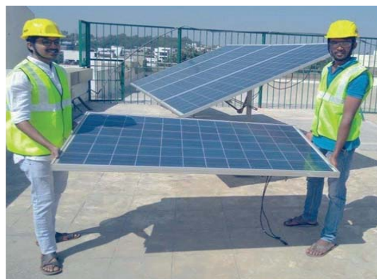
Solar technicians handling panel for next set of mounting. (Fig 3)
