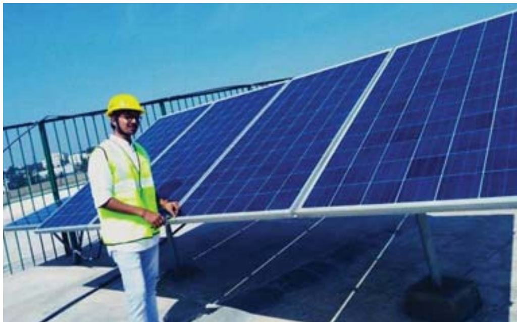
Solar panels 4 x 250 W mounted on mounting structures. (Fig 2)
