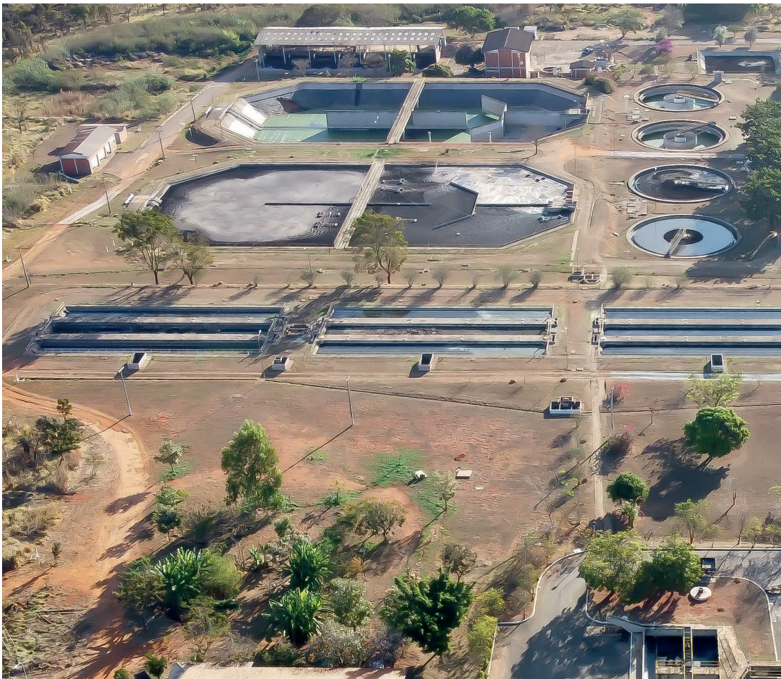
WWTP plant Gama in Brazil – an example of a 5-stage Bardenpho process for the removal of organic matter, nitrogen and phosphorus (photo: G. Da Luz Lima Júnior).
