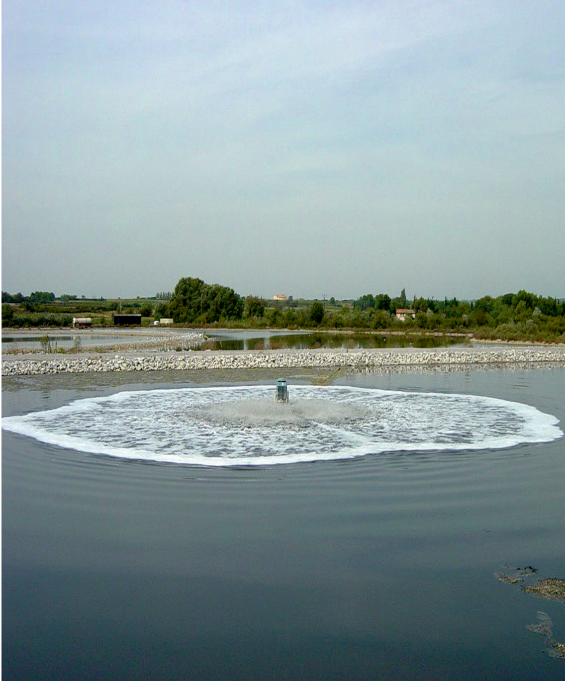
Aerobic lagoons and ponds are in many low- and medium-income countries prevailing technologies for the removal of organic matter from sewage, and faecal and septic sludge, often in combination with anaerobic and facultative ponds (photo: M. von Sperling).
