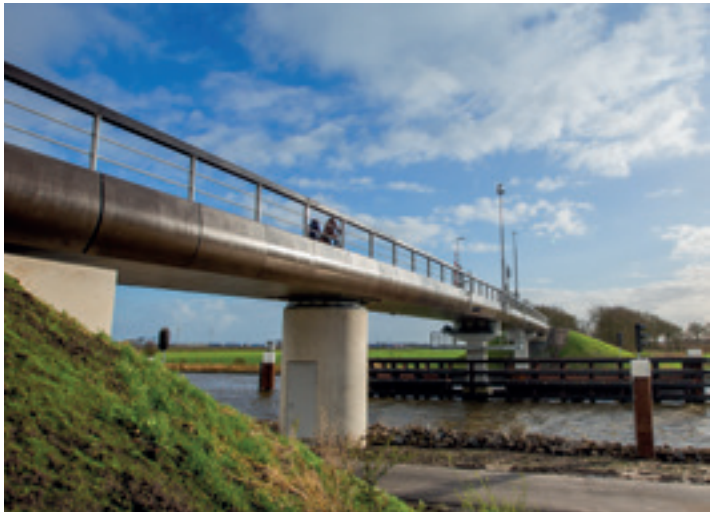
In the northern province of Friesland, a movable cycling bridge is being built with two decks made entirely from biocomposite (100% flax fibres and 80% bio resin): a world first at this scale.
