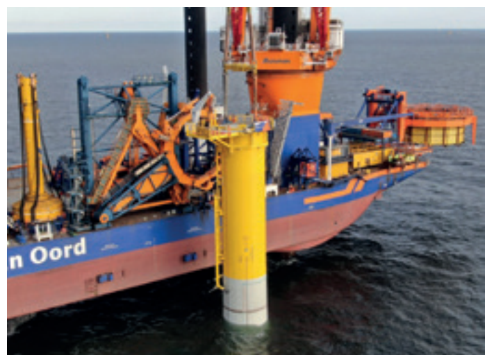
The Borssele Wind Farm Zone consists of 5 sites, one of which has been designated as an innovation site. In addition to the maintenance-free slip-joint method for connecting the monopile and transition piece, innovations include a new coating technology, eco-friendly scour protection, a new type of cable entry hole and a new ICCP monitoring system.
