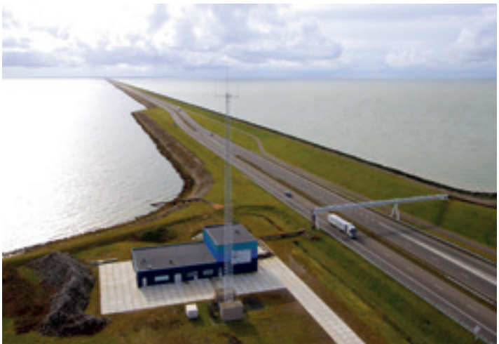
The Afsluitdijk dam separates the Wadden Sea from Lake IJssel, the Netherlands' largest freshwater reservoir. Dutch company REDstack built a pilot plant which generates electricity from the difference in salt content on either side of the dam, using reverse electrodialysis.
