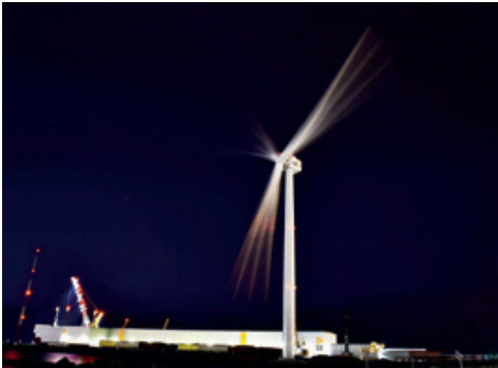
GE is currently building and testing the world's largest wind turbine, on the North Sea coast near Rotterdam, in close cooperation with ECN part of TNO. The Haliade-X turbine is 260 metres high, with 107-metre-long blades, and has an unprecedented capacity of 12 MW: enough to deliver electricity for 16,000 households.
