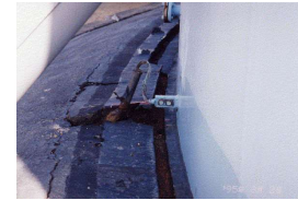
(e) Pulled out of earthing wire
