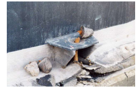
(b) Cut off of anchor bolt
