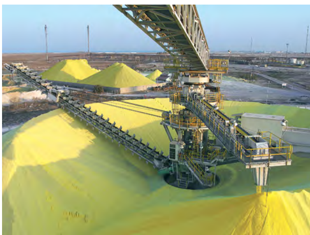
Figure 3. Circular stacker reclaimer for storage of solid sulfur pastilles.
