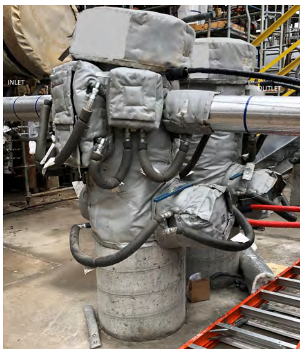
Figure 4. Sulfur seal with zero elevation change from inlet to outlet.
