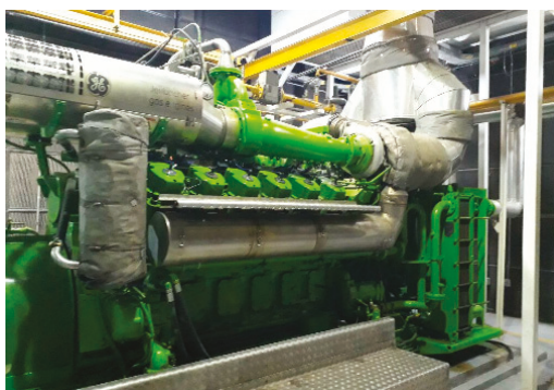
Figure 1. Jenbacher JMS-612 GS-N. L natural gas engine.
