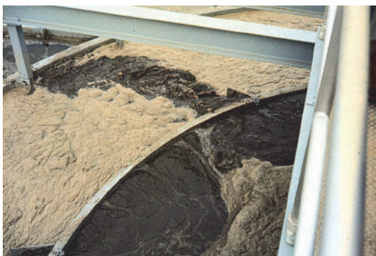
Figure 12.8 Scum on a clarifier (photo: Black and Veatch).
