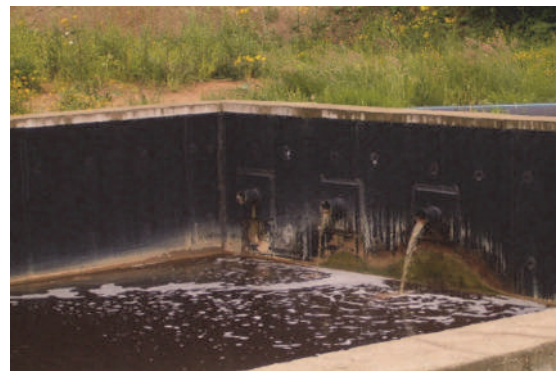
Figure 3.12 Collection and storage of leachate at a sanitary landfill site in Sarajevo in Bosnia and Herzegovina (photo: F. Babić).
