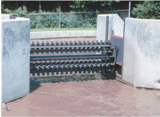
Figure 9.10 An oxidation ditch (shown schematically above) equipped with a surface brush aerator during standby (bottom left) and in operation (bottom right). The aerator's shaft is mounted on rails that can adjust the power drawn and lift the entire aerator above the free water surface, thereby avoiding any obstruction to the liquid flow.
