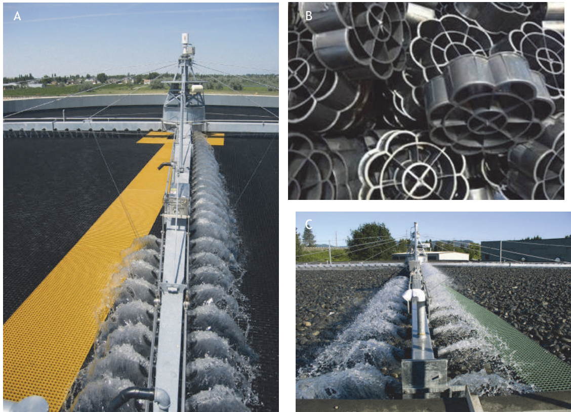
Figure 18.3 Trickling filters using (A) structured plastic, (B) random plastic or (C) rock as the biofilm support medium (photos: WesTech Engineering Inc. and Raschig USA Inc.).
