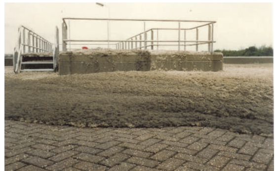
Figure 10.11 Extreme manifestation of sludge bulking (photos: Eikelboom, 2006).
