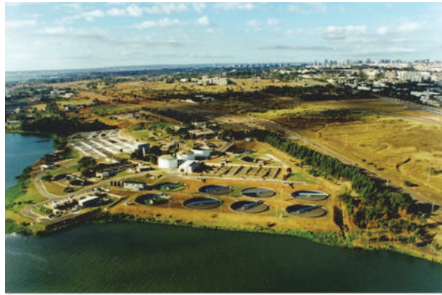
Figure 4.15A One of two wastewater treatment plants in Brasilia, Brasil (photo: R. Brummer).
