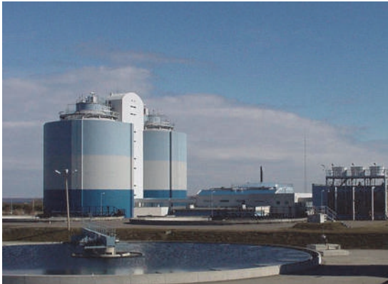
Figure 3.13 Digesters produce digester supernatant which often gives rise to problems in wastewater treatment plants due to the high loads of nitrogen and other substances (photo: D. Brdjanovic).
