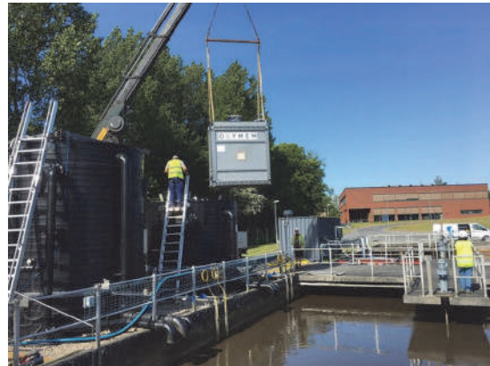
Figure 18.15 MABR module (photo: OxyMem).
