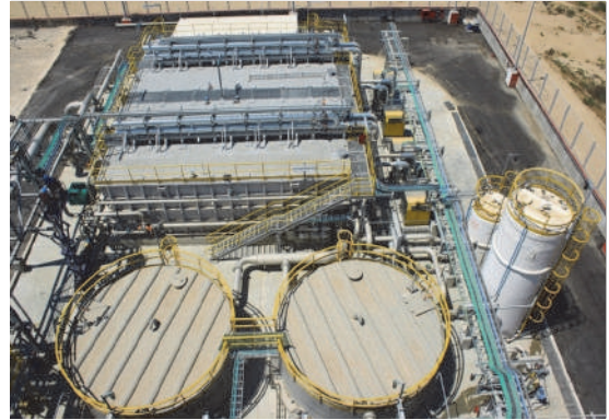
Figure 13.24 Aerial view of the MBR treatment plant belonging to Adama Agan Ltd.
