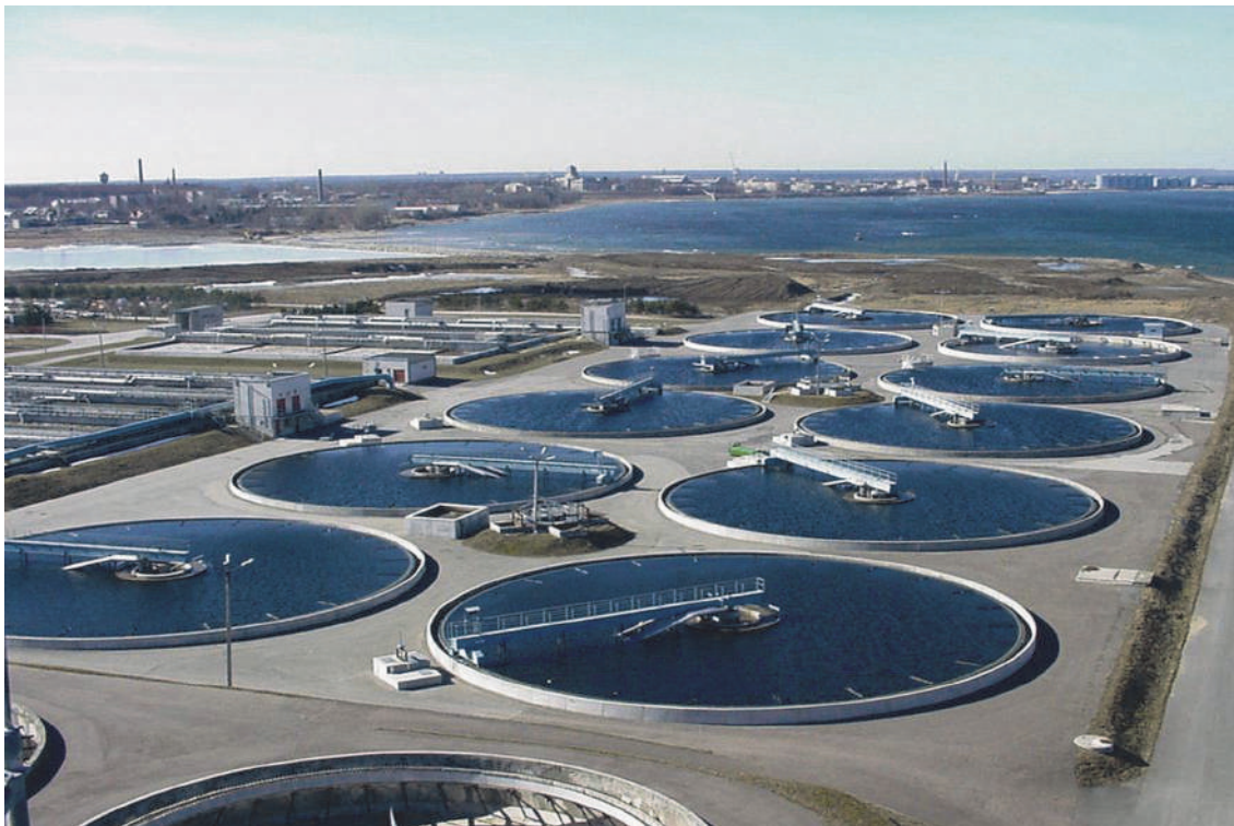
Figure 12.1 Final settlers are one of the most visible structures on Earth from space (photo: D. Brdjanovic).
