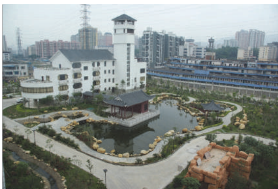
Figure 13.20 Aerial view of the Jingxi WWTP.
