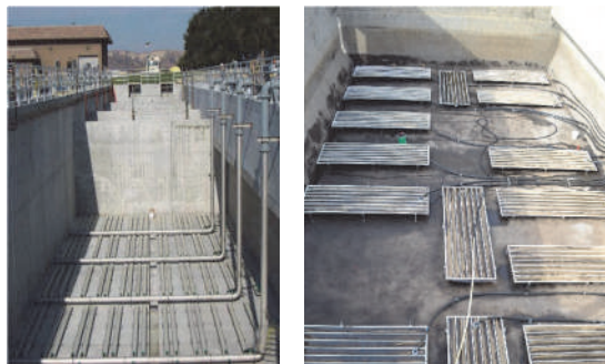
Figure 9.6 Examples of full-floor installations of fine-pore diffusers. Top: ceramic discs; bottom left: polyurethane strips; bottom right: polyurethane panels.
