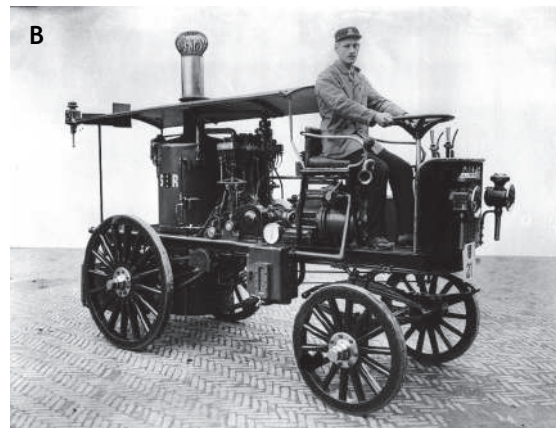
Figure 1.1 The Liernur vacuum sewer system (A) and the vehicle used for collection and transport of waste (B) (photos: Van Lohuizen, 2006).
