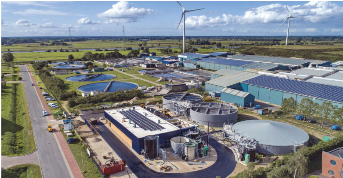
Figure 11.17 The Nereda ® plant in Zutphen, the Netherlands with a Kaumera-extraction plant. In the background is the existing conventional activated sludge plant.
