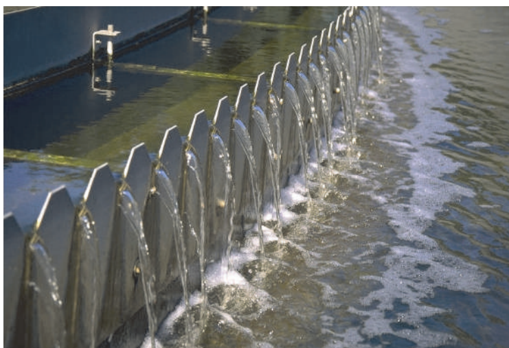
Figure 12.33 Example of properly operated and maintained secondary settling tank which produces effluent of good quality (photo D.H. Eikelboom).
