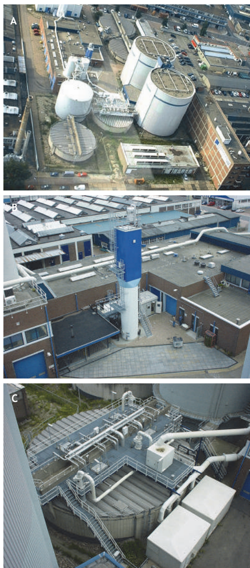
Figure 5.30 (A) Aerial view of sludge treatment facilities at the WWTP Dokhaven and view of the ANAMMOX® (B) and SHARON® (C) reactors taken from the top of the sludge digester (photo: Water Board Hollandse Delta).
