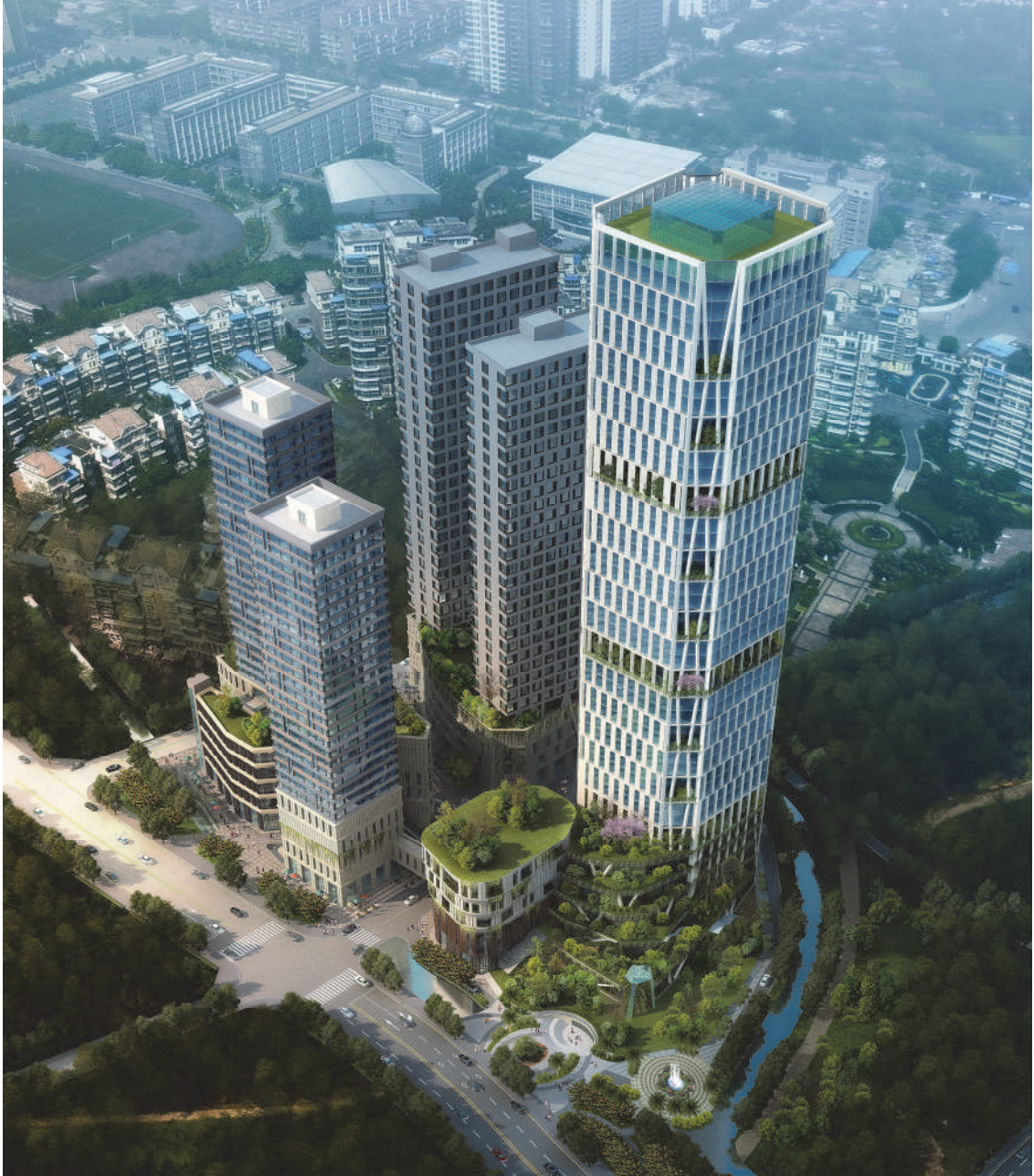
Figure 13.35 Hospital buildings in Guiyang, China have an underground, 50,000 m 3 /d, MBR plant for wastewater reclamation constructed 30 m beneath them (photo: G. Chen with courtesy of SEI and SUKE).
