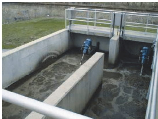
Figure 10.7 Aerobic selector (photo: M. van Loosdrecht).
