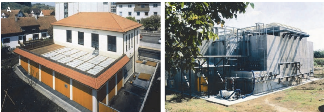
Figure 16.18 UASB installations for treatment of (A) fruit juice factory wastewater in Bregenz, Germany and (B) dairy wastewater in Indonesia (photos: Paques B.V. and Biothane B.V., respectively).
