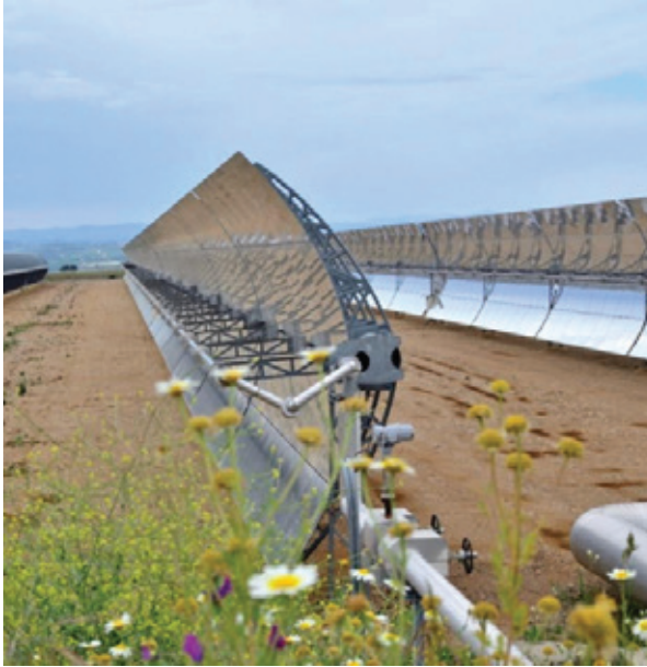
FIGURE 1.9 La Africana parabolic trough plant in Córdoba, Spain
