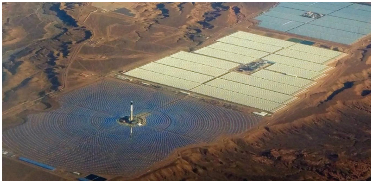
FIGURE 3.2 Noor Ouarzazate Solar Complex
