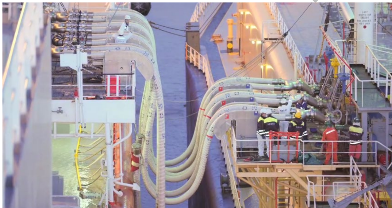
Figure 4-4 Flexible cryogenic hose system used in a side-by-side transfer configuration. [Source: The still taken from the Excelerate video]
