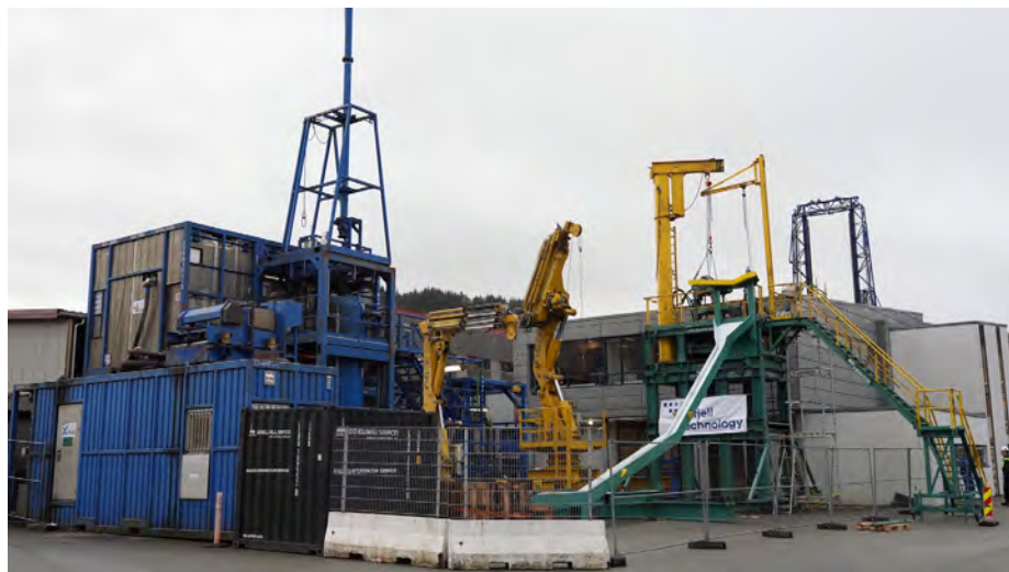
Figure 1. Rigless P&A unit.
