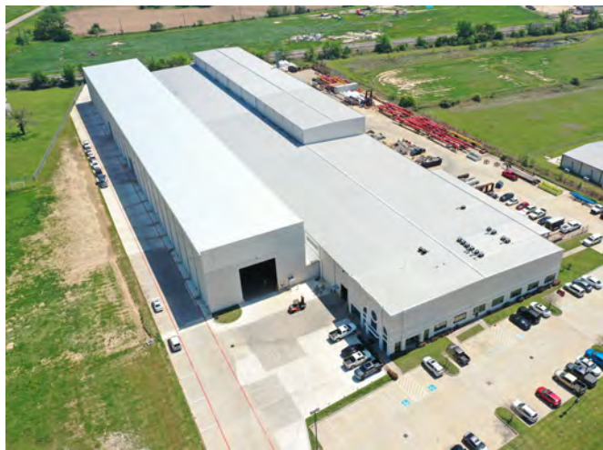
Figure 2. Logan Industries' manufacture and repair facility located in Hempstead, just outside of Houston, Texas.
