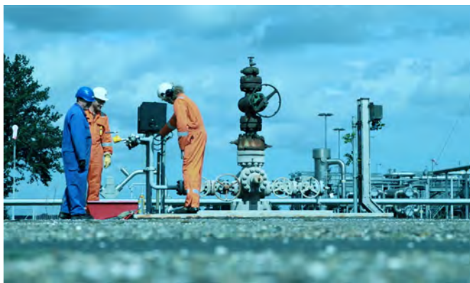
Figure 1. Installation of a HiberHilo sensor.
