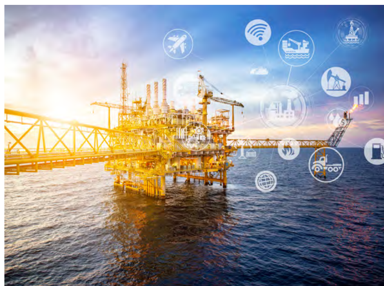
Figure 1. Utilising satellite technology can help operators deploy strong network connectivity to the most remote of sites.
