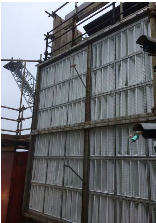
Figure 1. An offshore filterhouse undergoing an upgrade.
