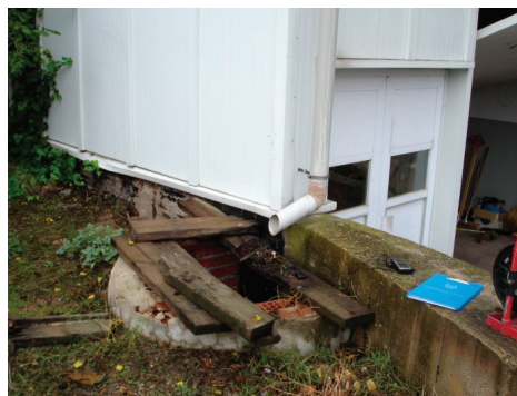
Figure 7. Example of a “very low cost” domestic MAR device in Madrid.
