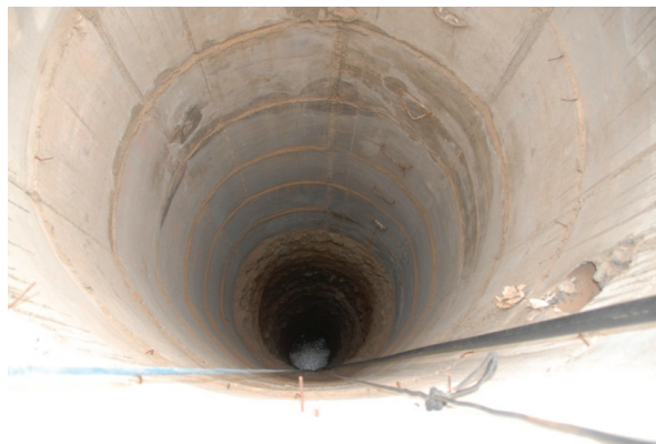
Figure 2. Two-meter diameter well showing the water level at about 20 m below surface in Wadi Qidayd, western Saudi Arabia.
