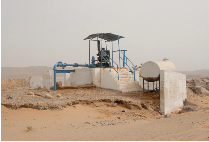
Figure 3. Abandoned municipal well that served a village water treatment facility.
