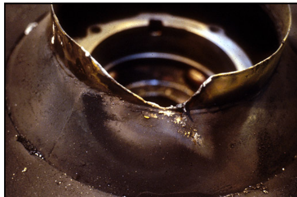
FIGURE 11: FAILURE OF AIR DEFLECTORS
