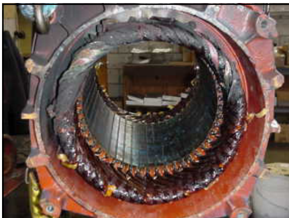
FIGURE 9: NONSYMMETRICAL THERMAL OVERHEATING
