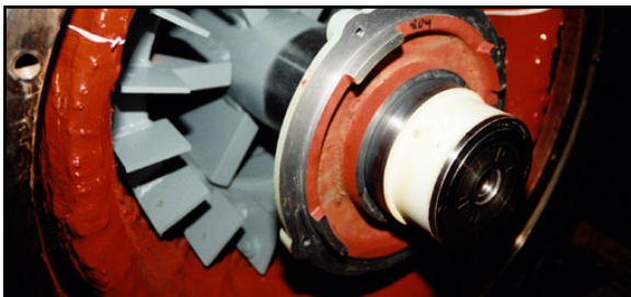
FIGURE 14: INSULATING WITH CERAMIC SPRAY
