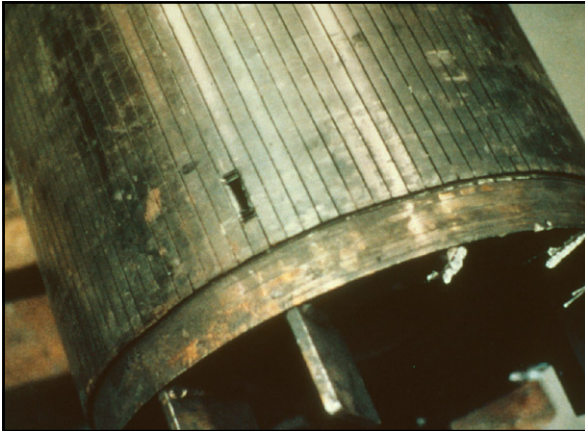
The rotor teeth fractured at the root due to resonance and were slung out into the stator, causing a ground failure.
