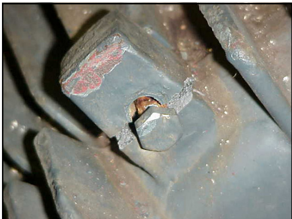
Due to excessive force, the ear cracked at the bolt circle.
