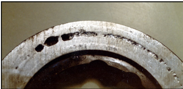
Voids located in an end ring.
