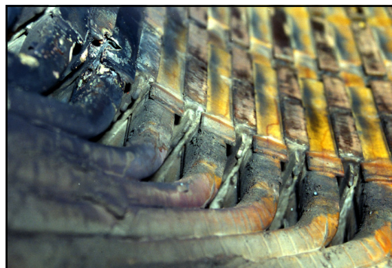
FIGURE 25: GROUND AT END OF SLOT
