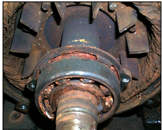
FIGURE 3: LUBRICANT DESTROYED BY THERMAL STRESS
