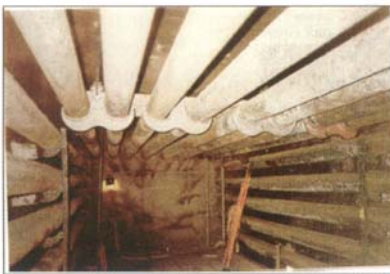
New roof hangers.
