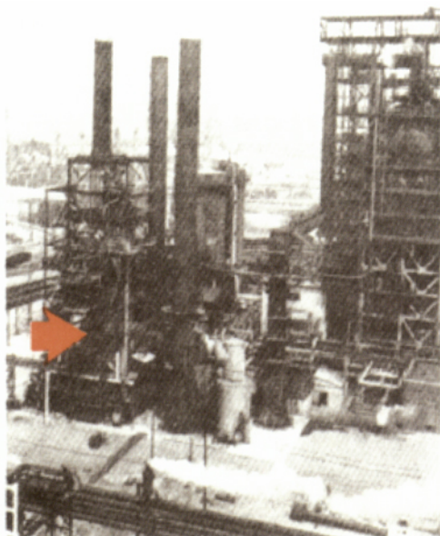
Figure 53 This waste-heat recovery operates under pressure to burn the carbon monoxide (CO) found in the flue gas of a catalytic cracker regenerator.
