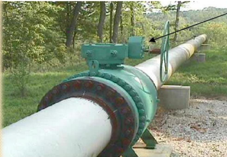
Actuator (handwheel and gearbox)
