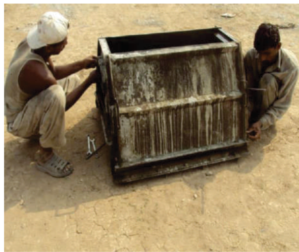
Assembling of Mold
