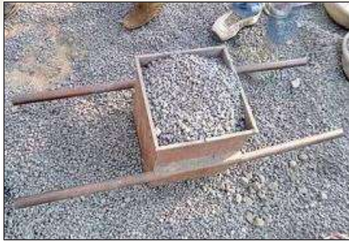
Figure-3.7 Use of measuring box for a batch of concrete
