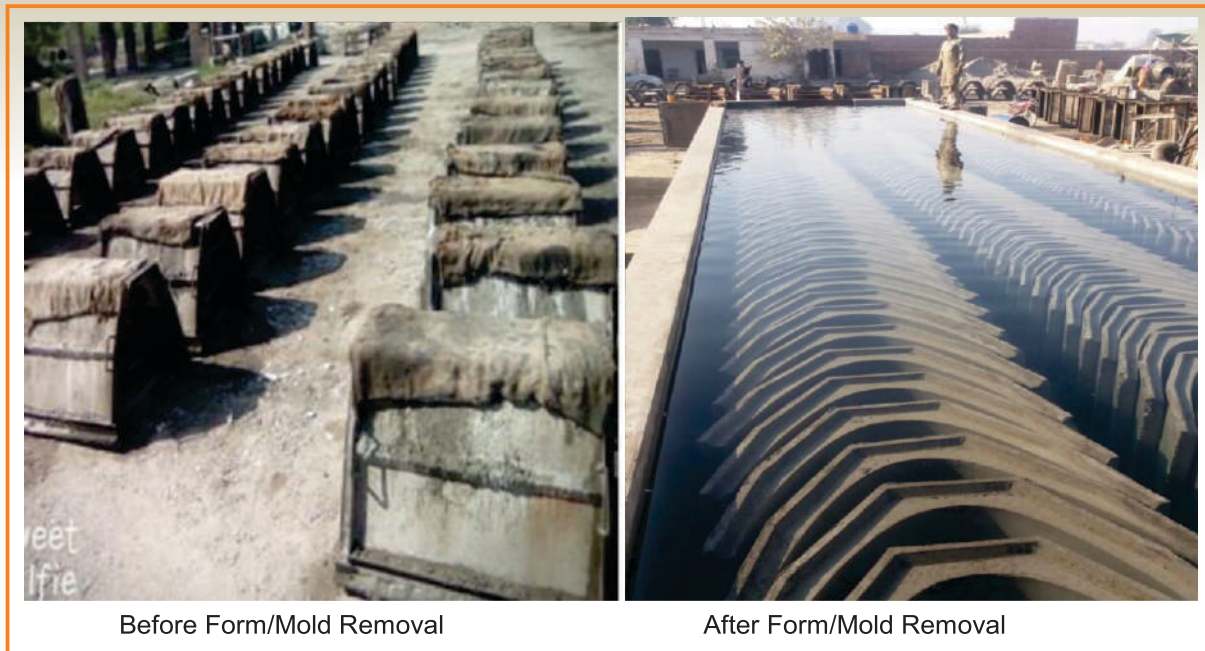
Figure-3.14 Curing of Pre-cast Concrete Parabolic Segments (PCPSs)
