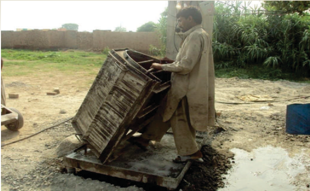
Concrete Placing on Vibrating Table
