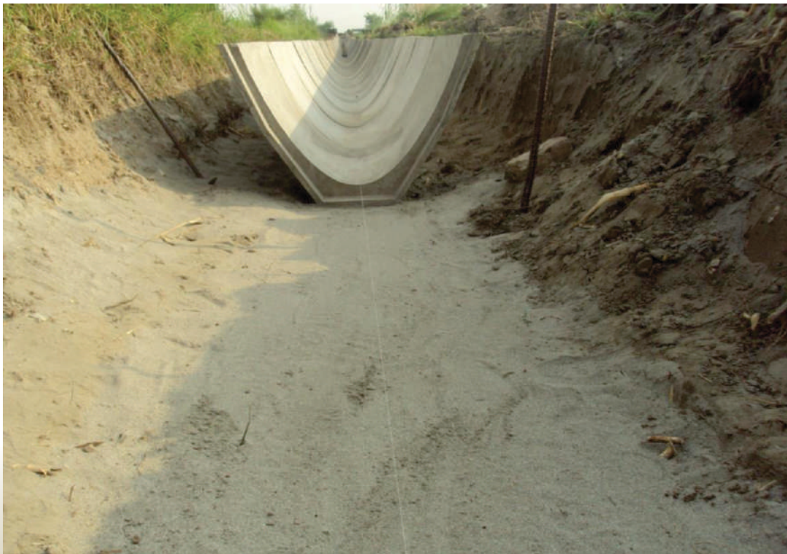
Figure-4.5 PCPS Installation Using String line
