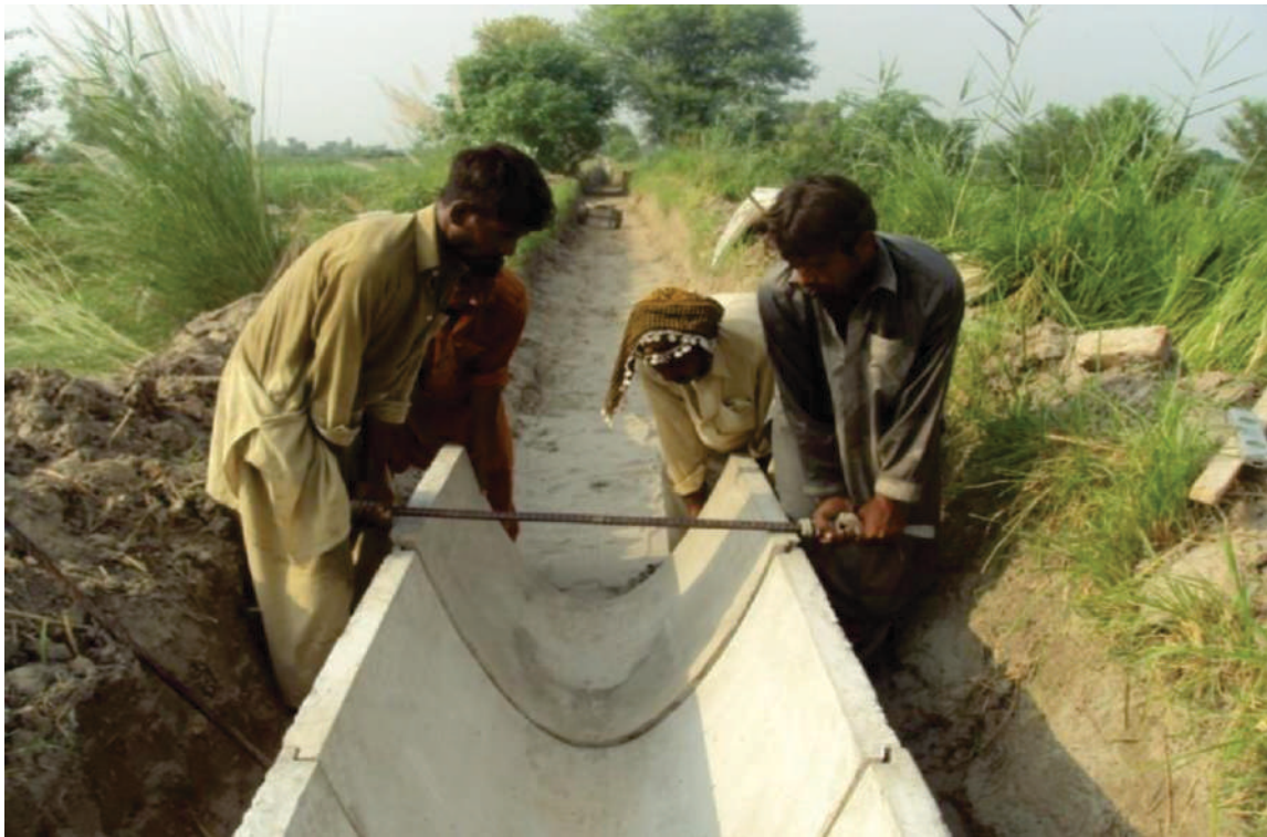
Figure-4.4a Placing PCPS in Position
