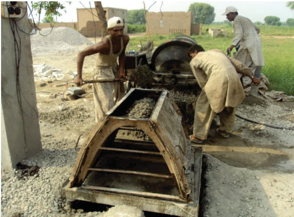
Figure-3.12 Setting Molds on Vibrating Table
