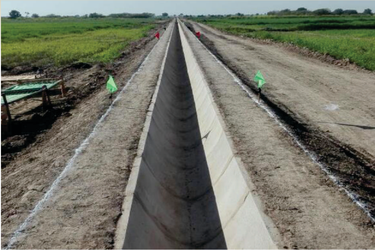
Figure-4.6 Finished Back Earth Filling
