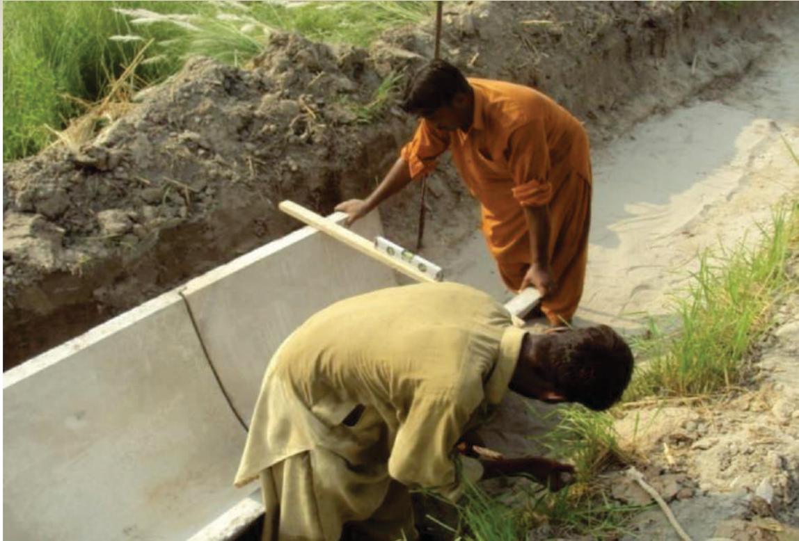
Figure-4.4b Checking and Adjusting PCPS for being in Horizontal Position
