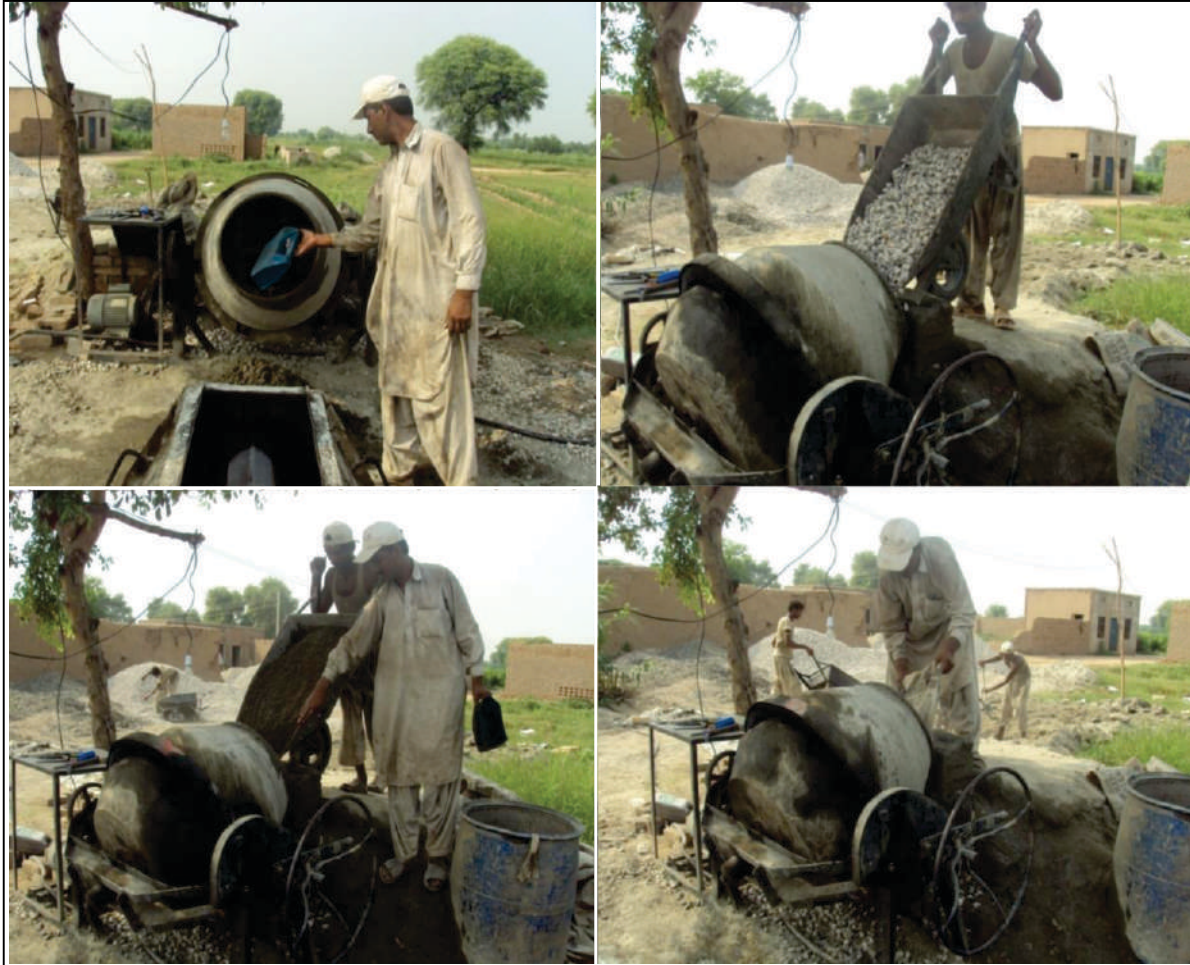
Figure-3.8 Pouring Material into the Mixing Machine
