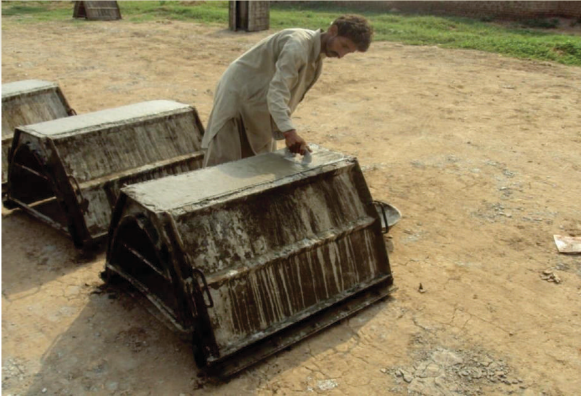
Figure-3.13 Fabrication of Precast Parabolic Lining Segment
