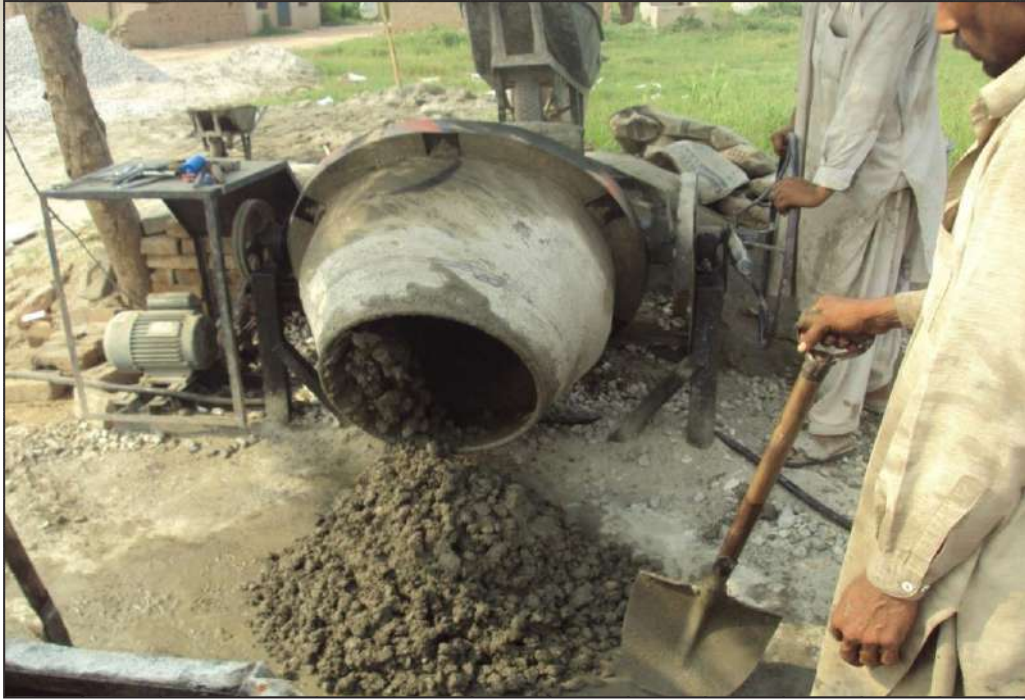
Figure-3.9 Concrete Ready for Placing in Molds
