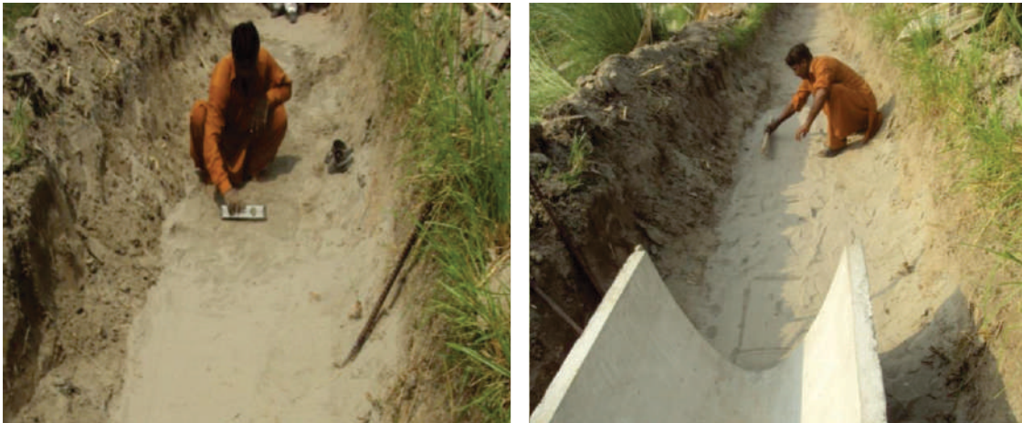
Figure-4.3 Sand Bed Preparation for PCPS Installation
