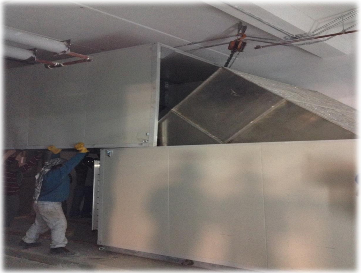
Plate Heat Exchanger AHU Site Construction and Installation
