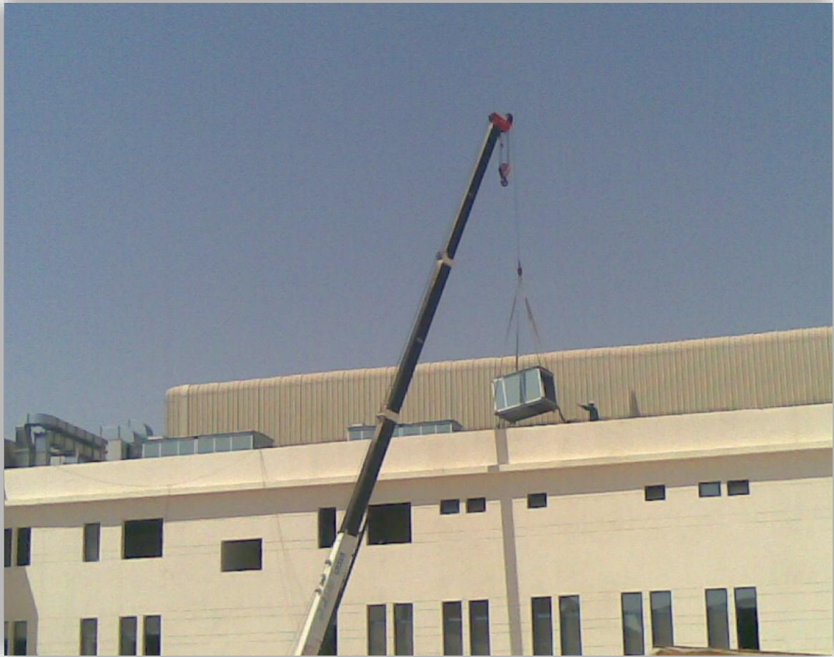
AHU Roof Site Installation
