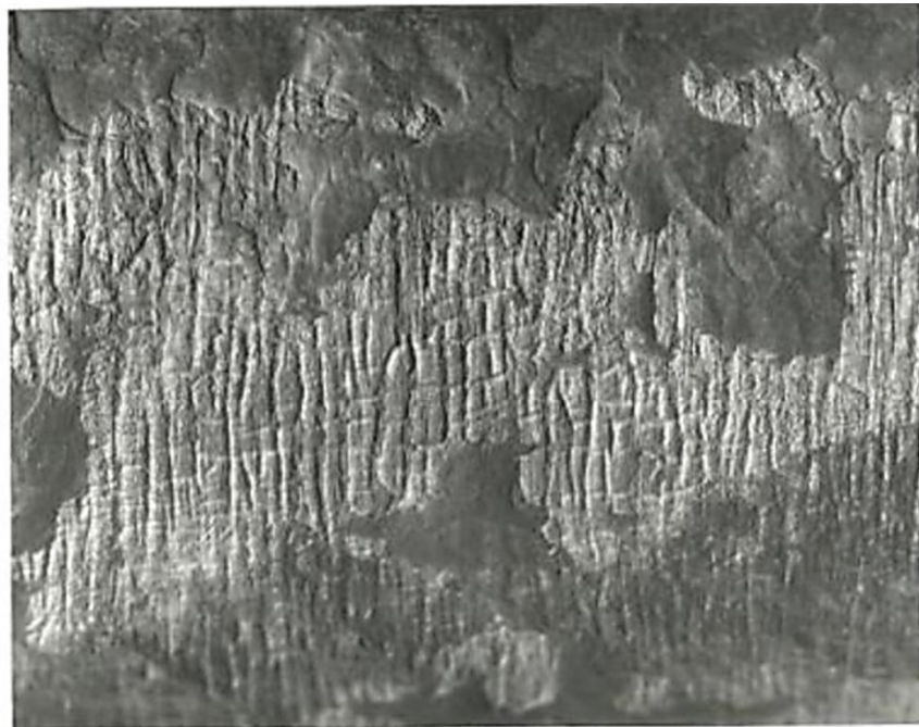
Figure 4-127 – The “alligator hide” morphology of liquid coal-ash corrosion is evident when the dense, glassy deposit is removed. Mag. 2.4X
