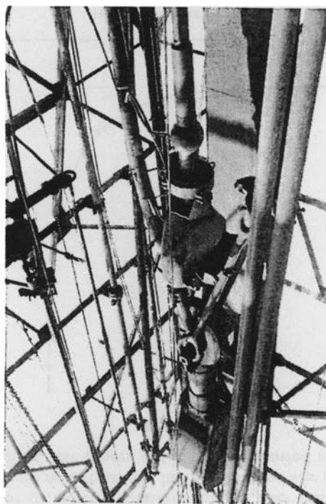
Figure 7.3 North Sea gas well drawgear—an IS instrumentation zone
