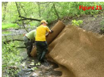
Erosion control blankets
