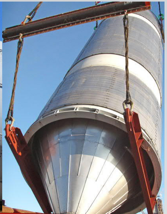
Tailing frame bolted to the skirt
