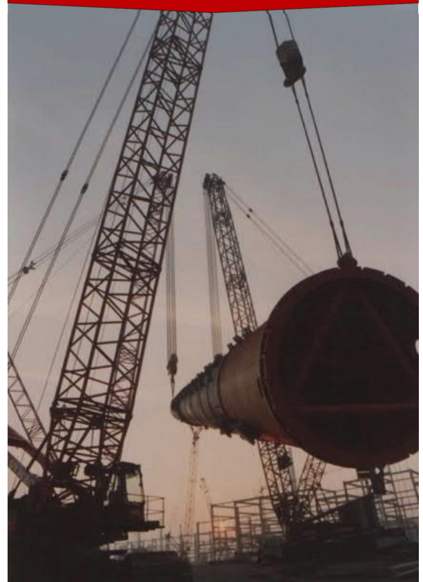
Lifting a 480 tons heavy column with 3 cranes
