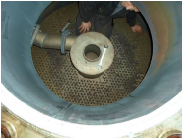
Figure 9: Top view central liquid inlet system
