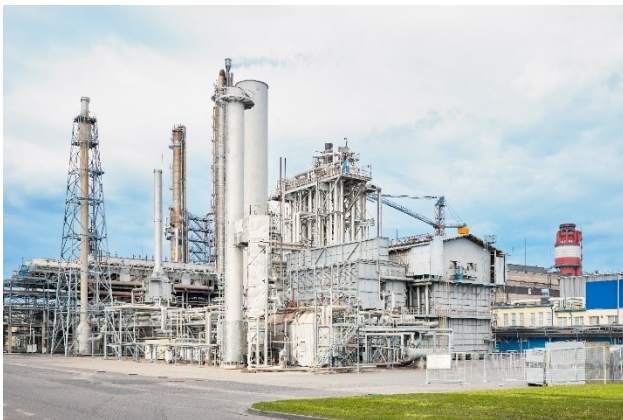
Figure 12. Ammonia plant site
