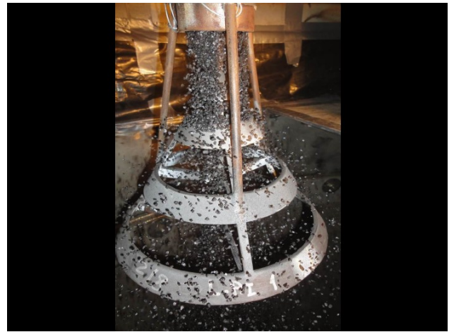
Figure 10. Catalyst distribution cone inside the catalyst bed (patented by thyssenkrupp Uhde)
