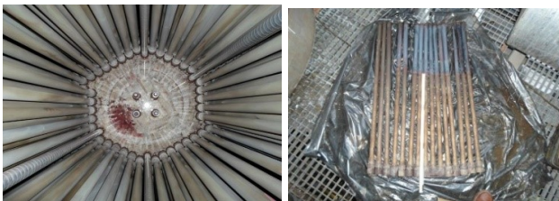
Figure 10: tubes centered around liquid inlet box flooded due to fluid retention.
