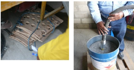
Figure 8. Time consuming filling of catalyst in layers of 30 cm (12 inch) via hose and vibrator
