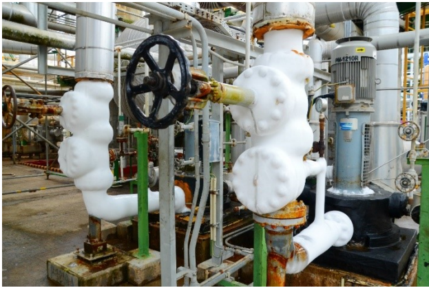
Figure 7. Cryogenic pumps
