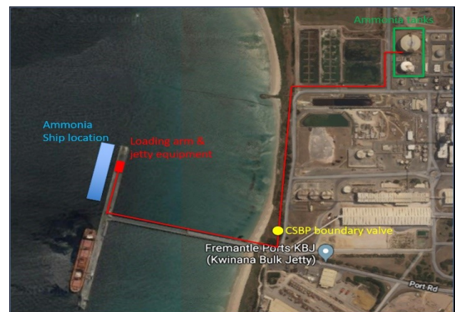
Figure 1. CSBP's ammonia loading facility at the Kwinana Bulk Jetty
