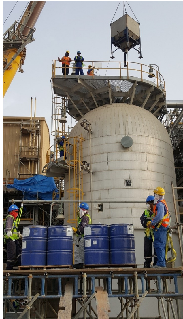
Figure 2. Catalyst loading process.
