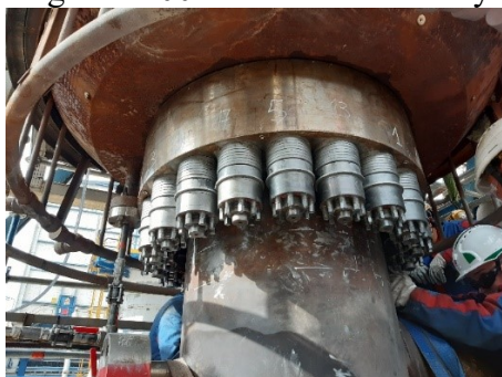
Figure 7. Repair activities in Synthesis Reactor
