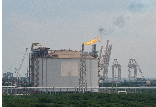
Figure 9. Storage tank flare
