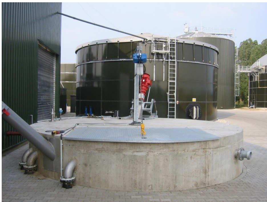
Figure 6.2: Storage for liquid feedstock (Fachverband Biogas e.V.)
