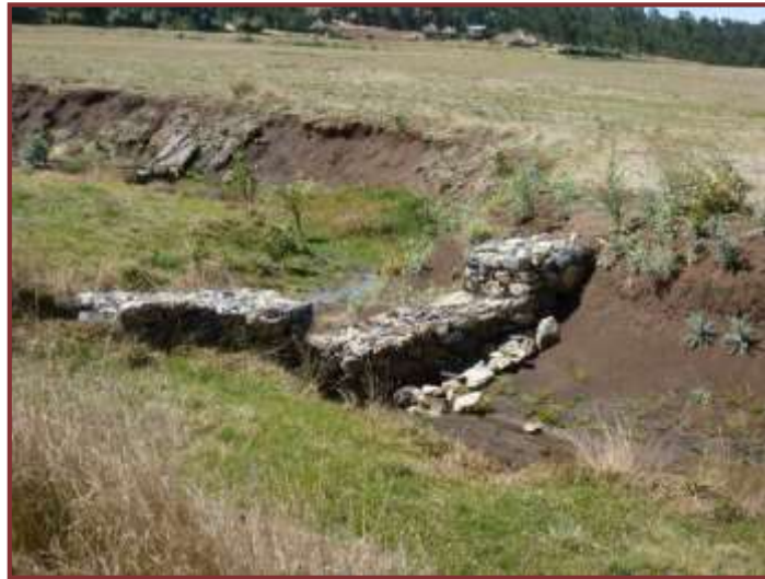
Figure A5: Photo of a reclaimed gully using check dams and re-vegetation
