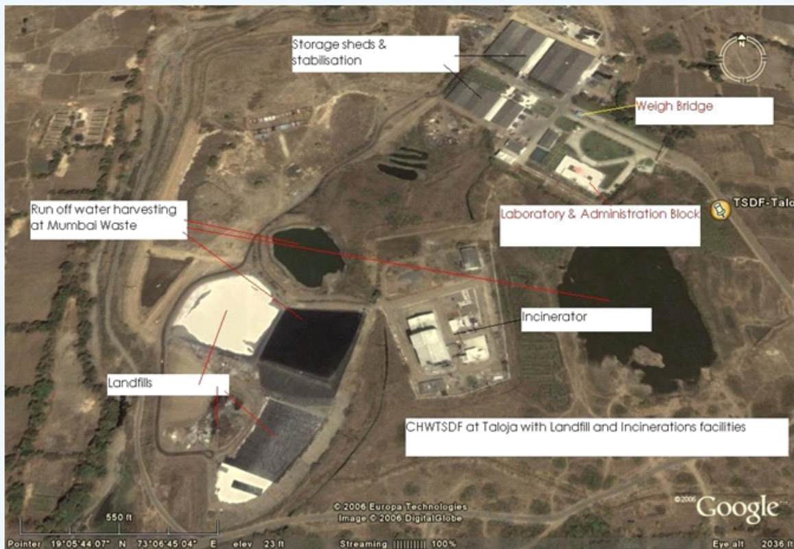
Figure – 7.2.2: An Aerial view of CHWTSDF at Mumbai
