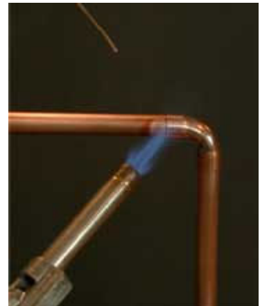
Figure 47: Soldering
