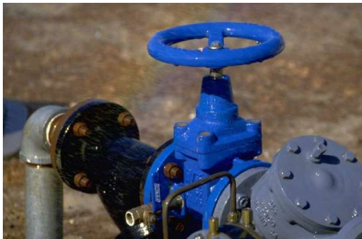
Figure 4: Valve and check valve
