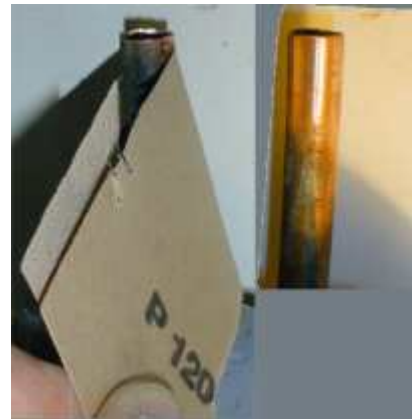
Figure 14: Cleaning the tube (2)
