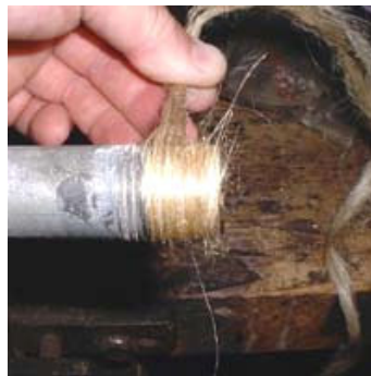
Figure 40: Applying oakum
