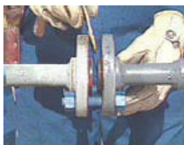
Figure 78: Installation of the bottom screws and the gasket
