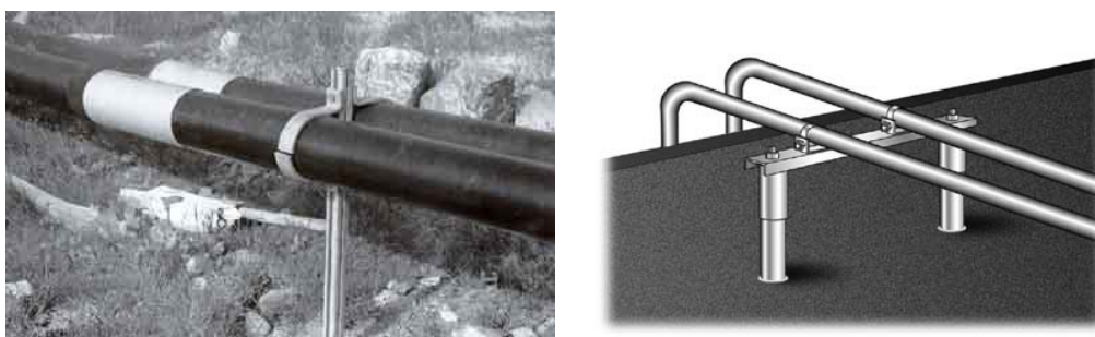
Figure 95: Support from underneath
