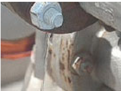
Figure 71: Leaking water pipe flanges
