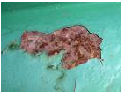
Figure 93: Rust penetration
