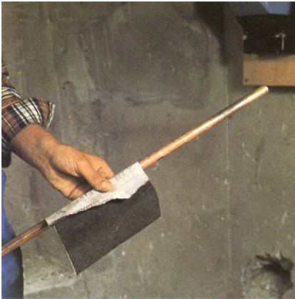
Figure 13: Cleaning the tube (1)
