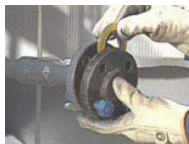
Figure 78: Installation of the bottom screws and the gasket
