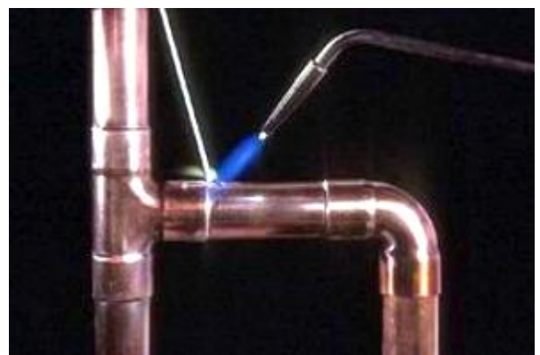
Figure 46: Soldering or brazing
