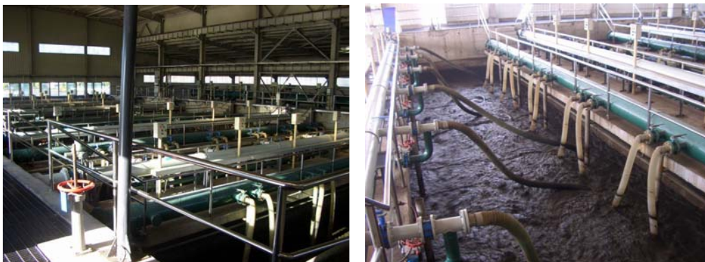
Figure 12. Photos of membrane tank in Miyun municipal wastewater MBR Plant, Beijing.
