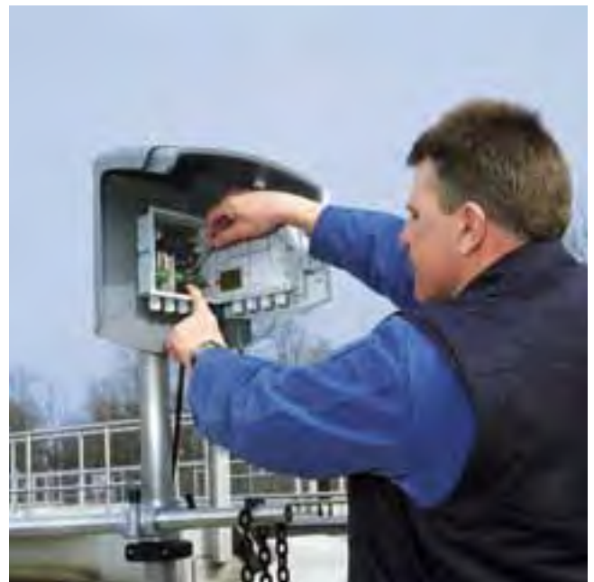
Simple installation at the process tank (on-site)
