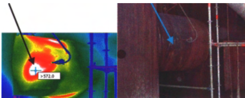
Figure 6.2.10. Refractory breakdown readily seen by white area in IR image.
