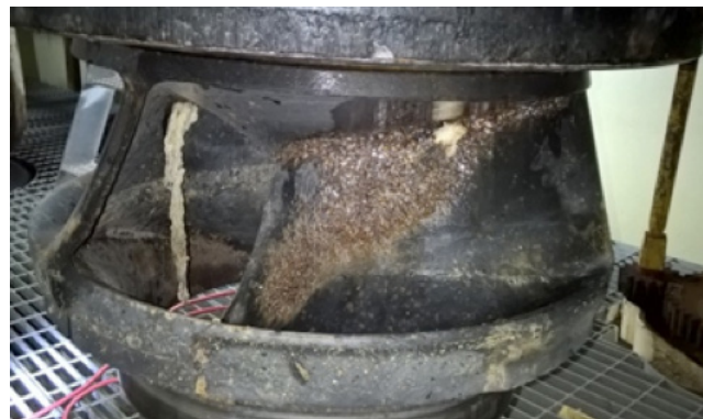
Figure 1: Cavitation damage on the blade of a centrifugal pump impeller.
