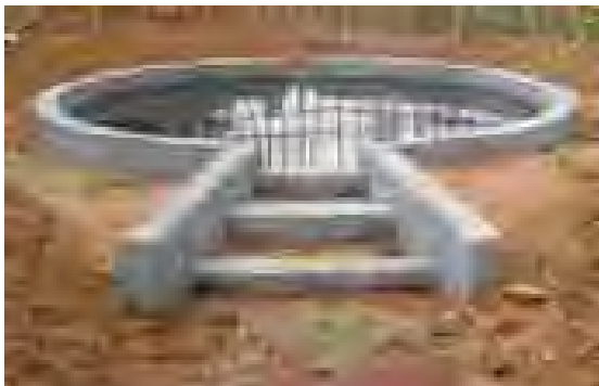
Figure 20. A completed rainwater-harvesting tank.
