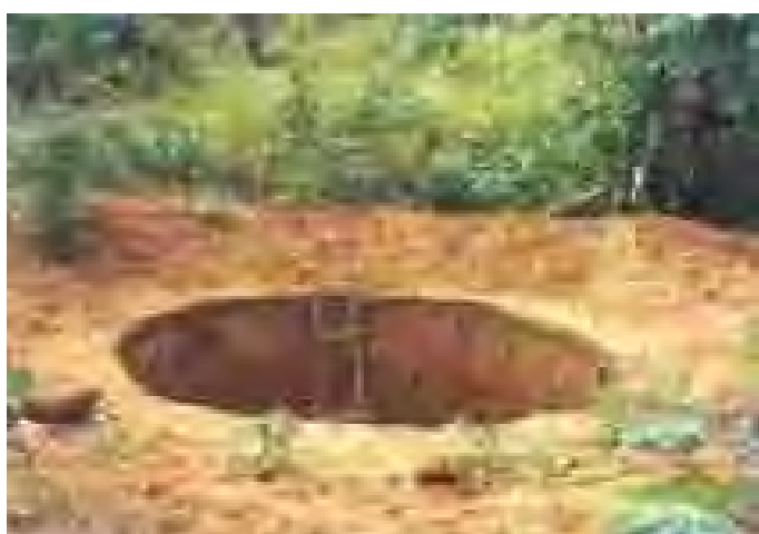
Figure 9. Pit for the tank construction.
