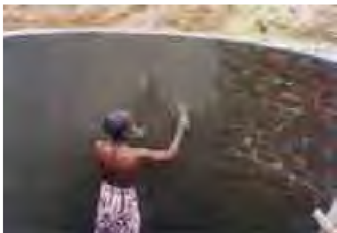
Figure 17. Plastering the tank.
