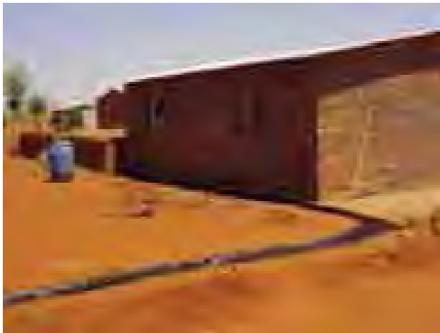
(b) Furrow alongside the house to divert water falling from the roof into underground tank.
