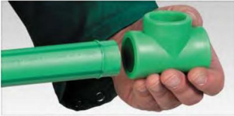
Aligning the fitting.
