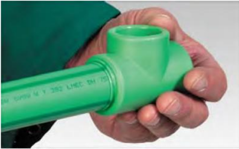
Joining the pipe.
