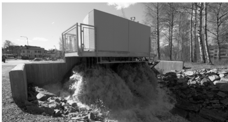
Figure 16. The Pietarsaari storm water pumping station.
