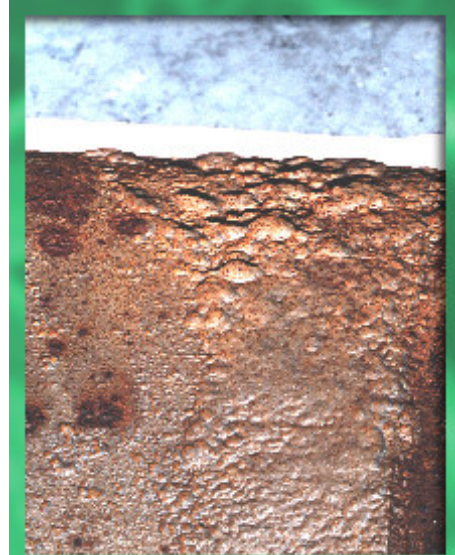
CO 2 corrosion of carbon steel
