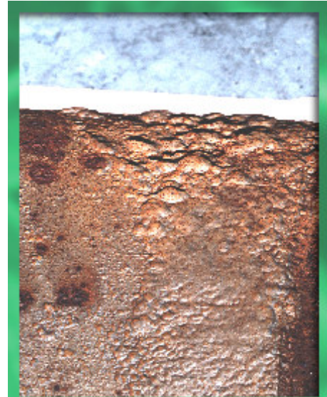
CO 2 corrosion of carbon steel
