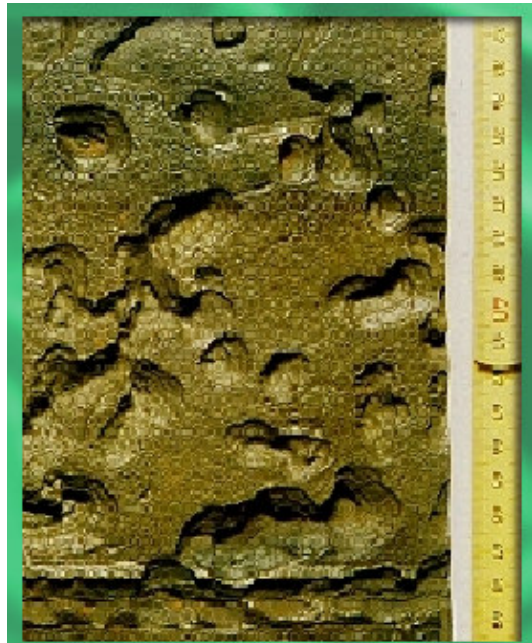
Carbon Dioxide Corrosion
