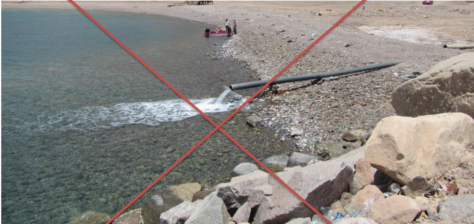
Old Brine Outfalls
