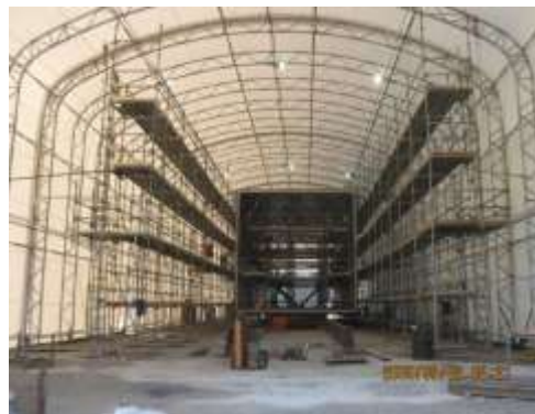
Figure 2 – This photo shows work inside the tent.
