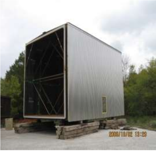
Figure 3- Insulated before raising into place
