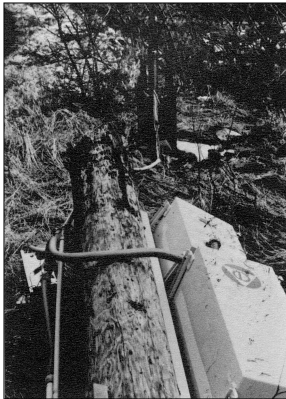
Figure 3-7 Downed pole-mounted transformer in Hurricane Iniki, Kauai, Hawaii
