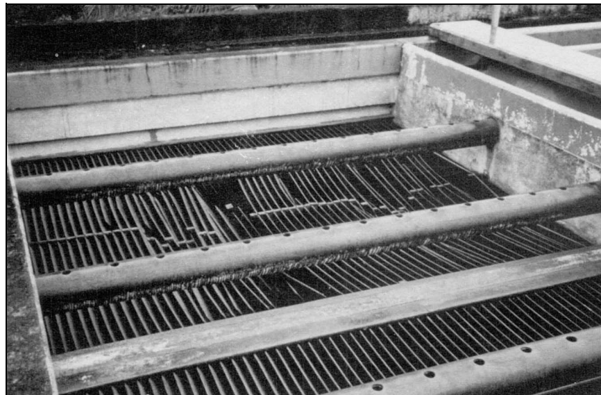
Figure 3-4 Damaged clarifier plates after earthquake in Limon, Costa Rica
