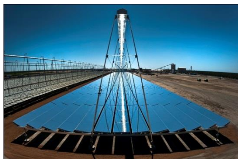
Fig 8.2 Fresnel lens
