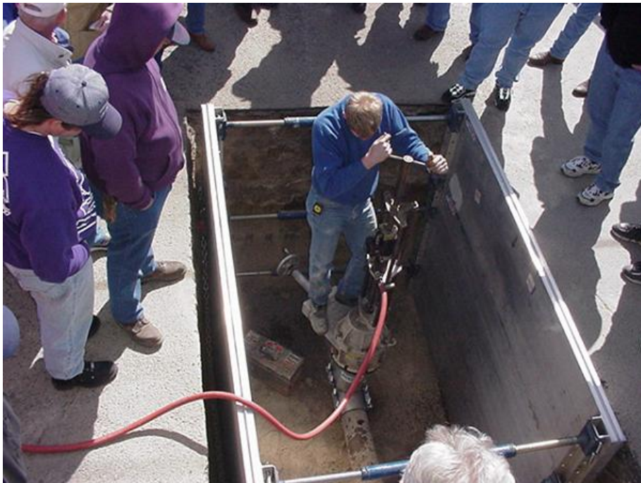
Hydro-stop valve insertion machine
