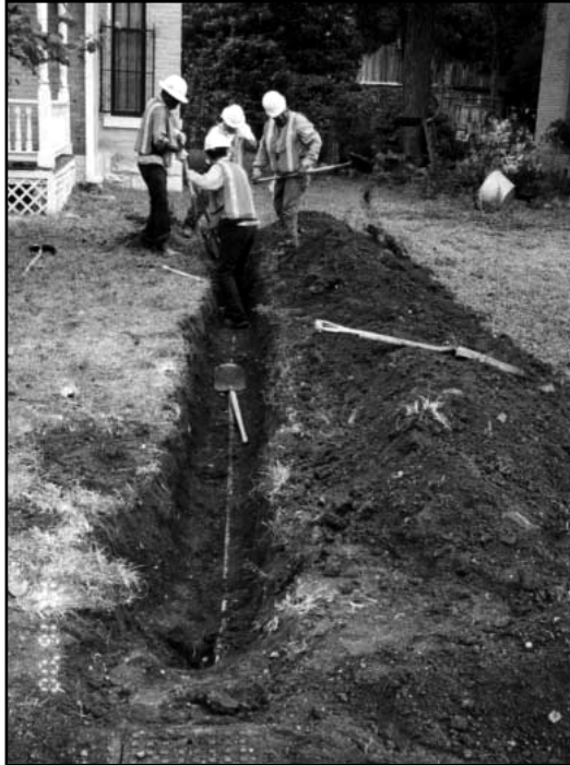
Figure 2 Collection of pipe samples from residential service line
