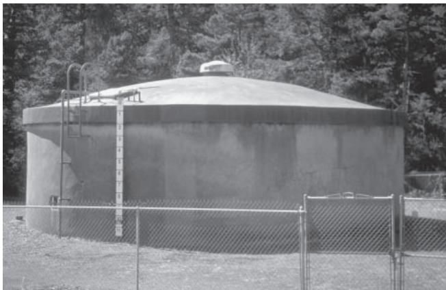
Water storage tank
