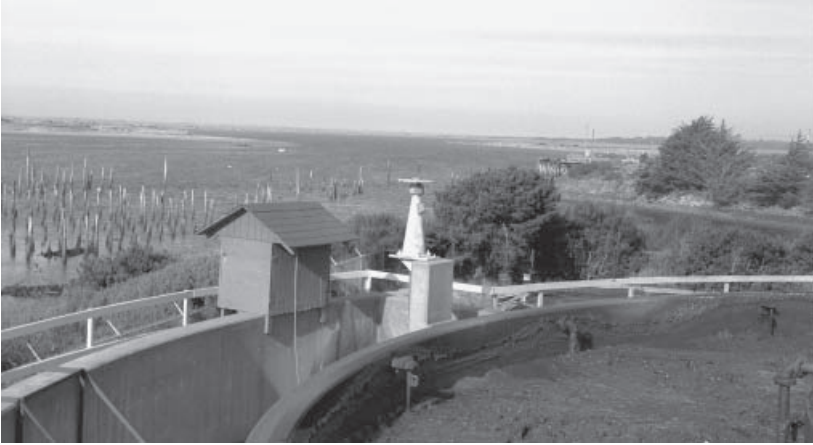
Municipal sewage treatment plant, Coquille Bay, Oregon
