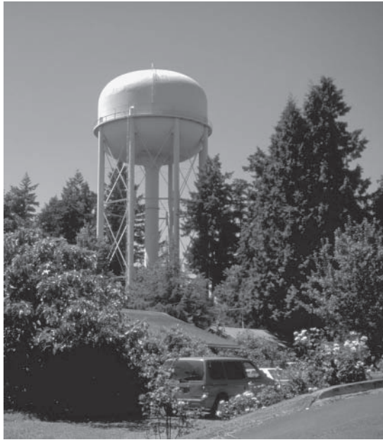
Water storage tower
