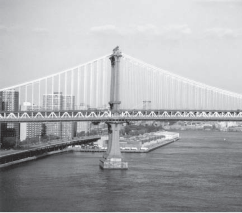
Manhattan Bridge and East River, New York
