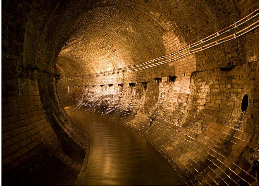
Brickwork sewer line
