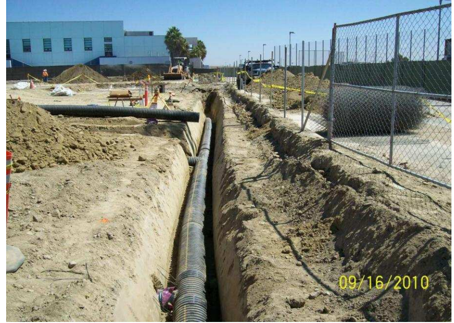
HDPE sewer pipe
