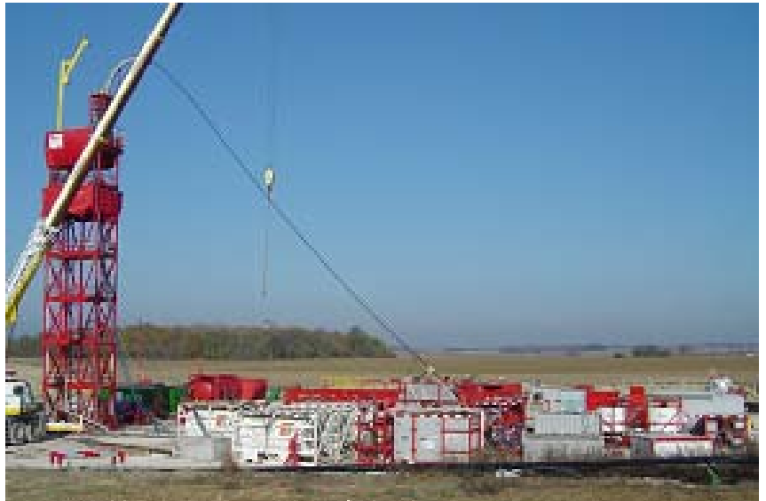
Figure 107 CTU Drilling Operation
