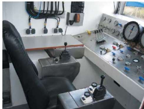
Figure 106 Zone II Control Cabin
