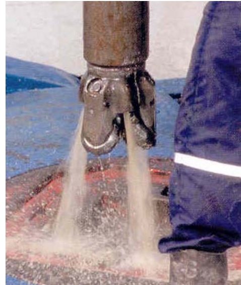
Figure 38 Mud Flowing through Bit
