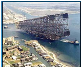
Figure 4 – Massive platform legs being towed into position
