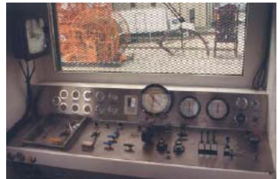
Figure 104 Inside a Control Cabin
