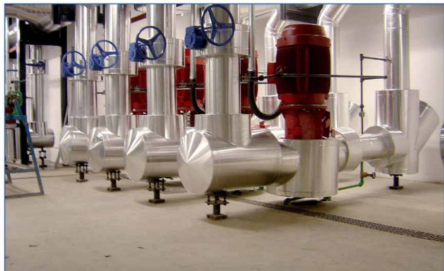
Figure 17 Vertical In-Line Pump (Single Suction Impeller)
