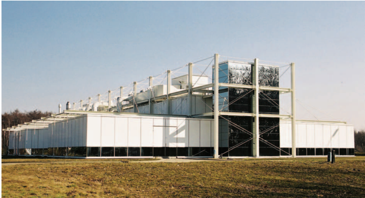
Figure 6 - Modern design of Welschap pumping station (Noord-Brabant) where anaerobic groundwater is treated to produce drinking water
