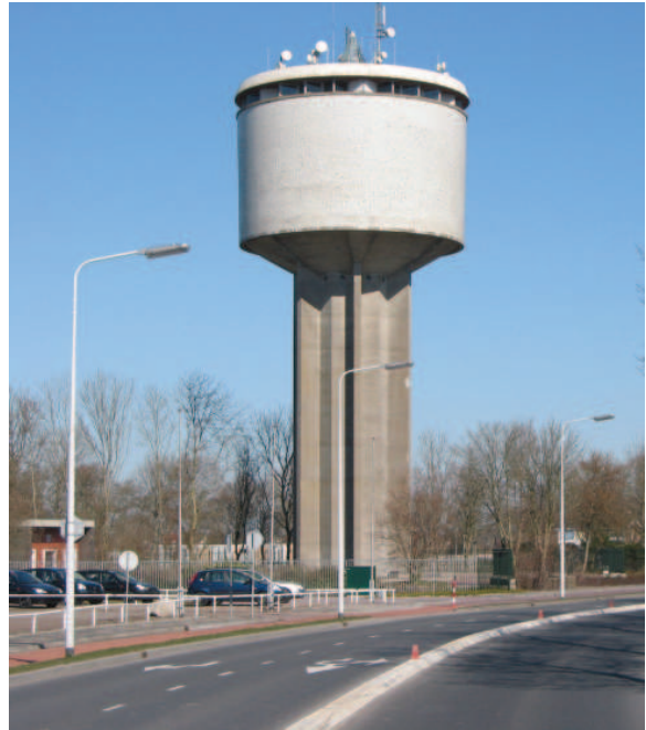
Figure 20 - Water tower in Dokkum
