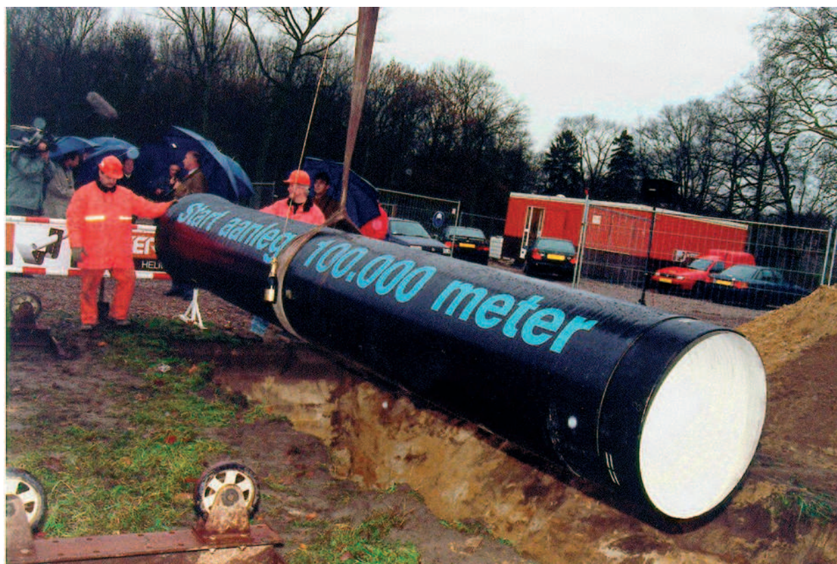
Figure 24 - For all alternatives, a considerable pipeline infrastructure was needed
