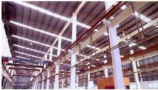
Figure 17. Day lighting with poly carbonated sheets
