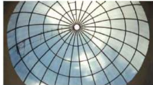
Figure 18. Atrium with FRP dome
