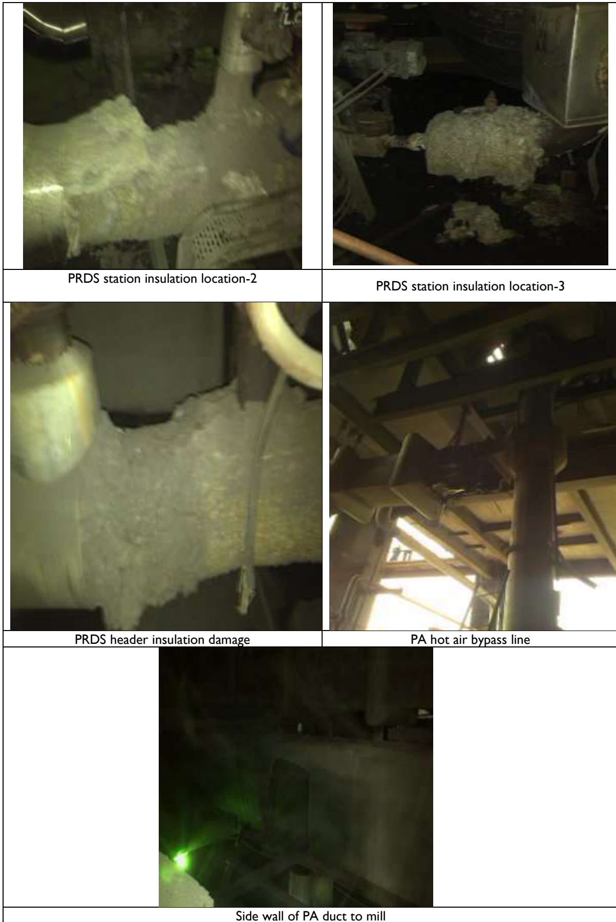
Figure A5-11: Images of evaluation of insulation condition
