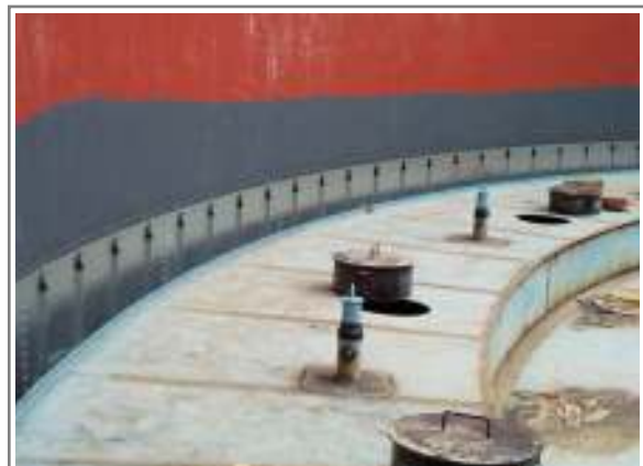
Shoe Plate after Installation
