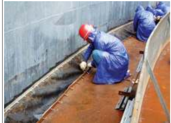
The installation of continuous seal (Tank Dia 60M-China oil company)
