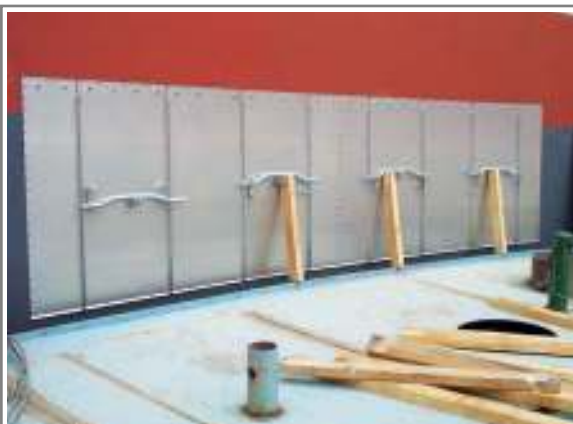
Shoe Plate before Installation
