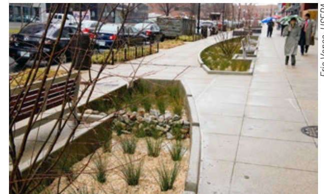
Bioretention cell in sidewalk with seating along a commercial corridor in Washington, DC.
