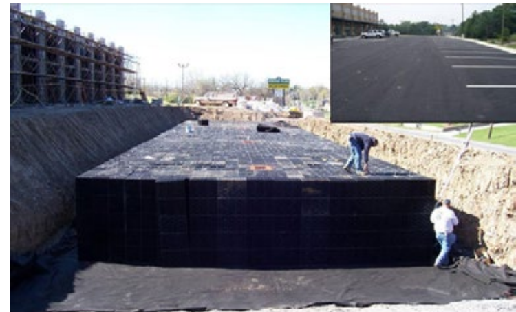
Subsurface chambers, during and after (top right) installation.
