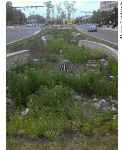
Figure 4-22. Beehive overflow grate prevents debris from entering the overflow structure in a roadside bioswale in Arlington, VA.
