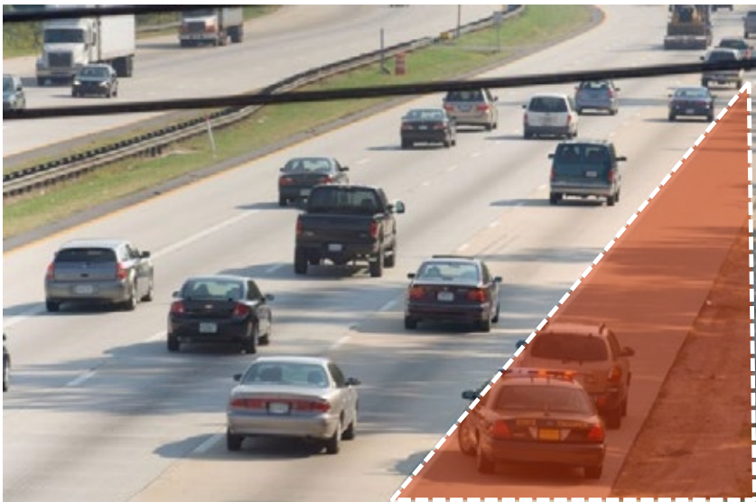
Figure 2-8. Green elements such as a swale, permeable pavement or a permeable friction overlay can be added in the verge area (roadside zone).
