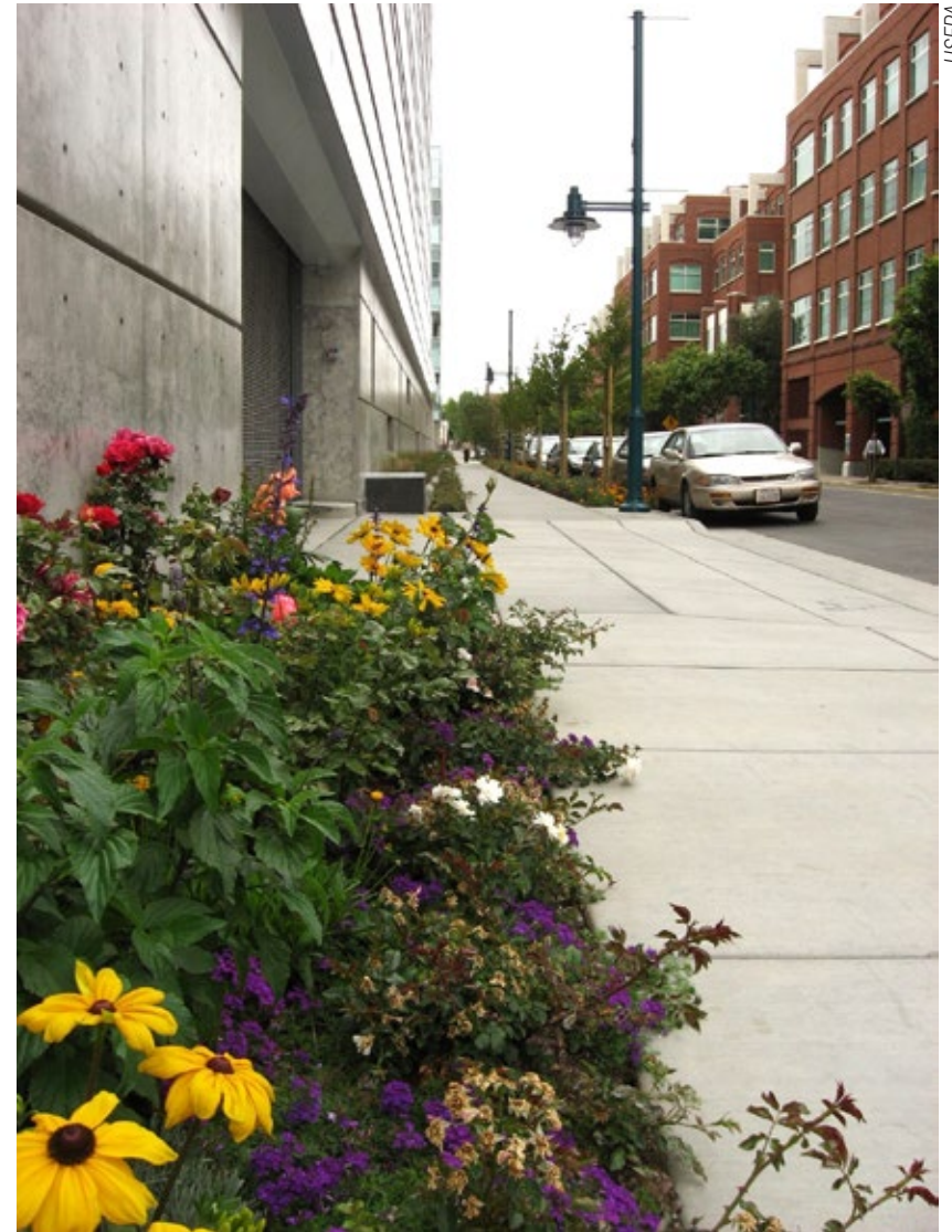
Sidewalk planters capture runoff from a local road in Emeryville, CA.
