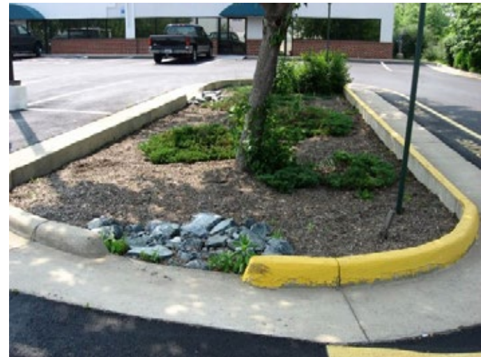
Figure 1-2. Modifying or designing parking lot islands as bioretention areas can capture and temporarily store runoff, allowing the water time to infiltrate the soil or be evapotranspired.
