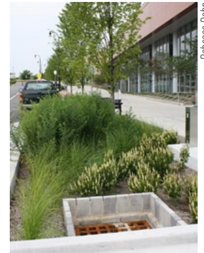
Figure 4-20. Concrete band structure constructed around the outflow allows ponding in Nashville, TN.
