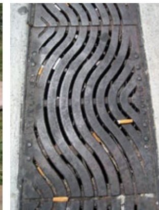
Figure 4-28. The small spaces in this grate are clogged with cigarette butts, which block drainage and are difficult to remove.
