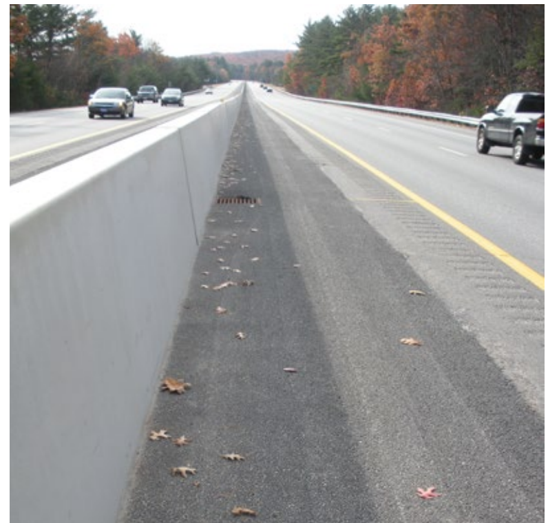
Permeable friction course on the shoulder of I-293 in New Hampshire.
