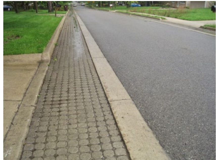
Permeable pavers used in the parking lane of a roadway in Ann Arbor, MI.
