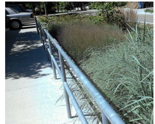
Figure 4-34. Fence protects pedestrians from the drop in grade in the adjacent bioretention feature in Minneapolis, MN.
