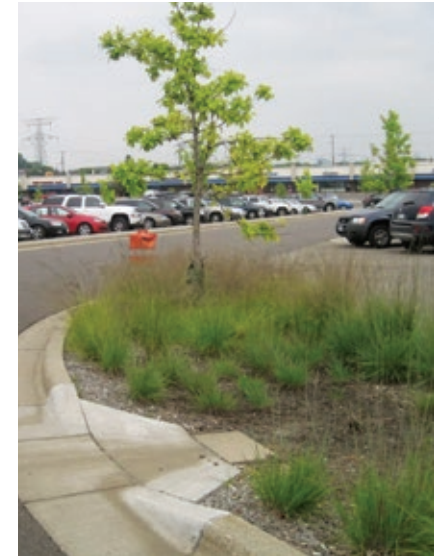
Figure 2-12. A parking lot island includes a bioretention feature in Maplewood, MN.
