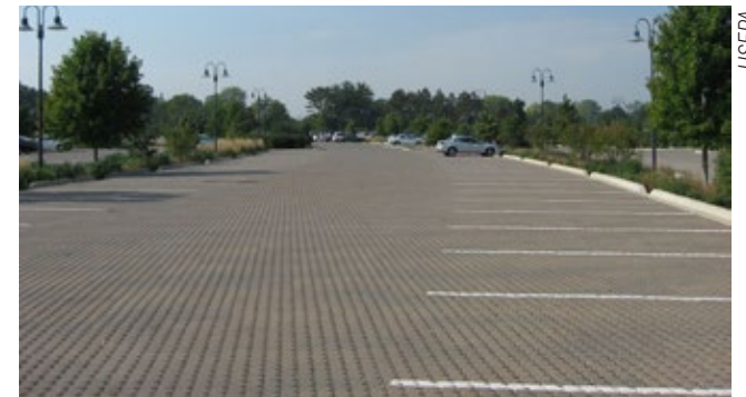
Permeable interlocking concrete pavement, Chicago, IL.
