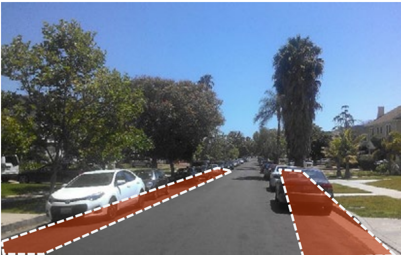
Figure 2-9. Alternative surfaces such as permeable pavement can be used in on-street parking lanes.
