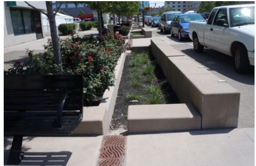
Interconnected stormwater planters include protective walls alongside the parking lane in Niagara Falls, NY.
