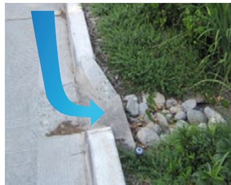
Figure 4-2. An angled curb cut with a graded gutter, Seattle, WA.
