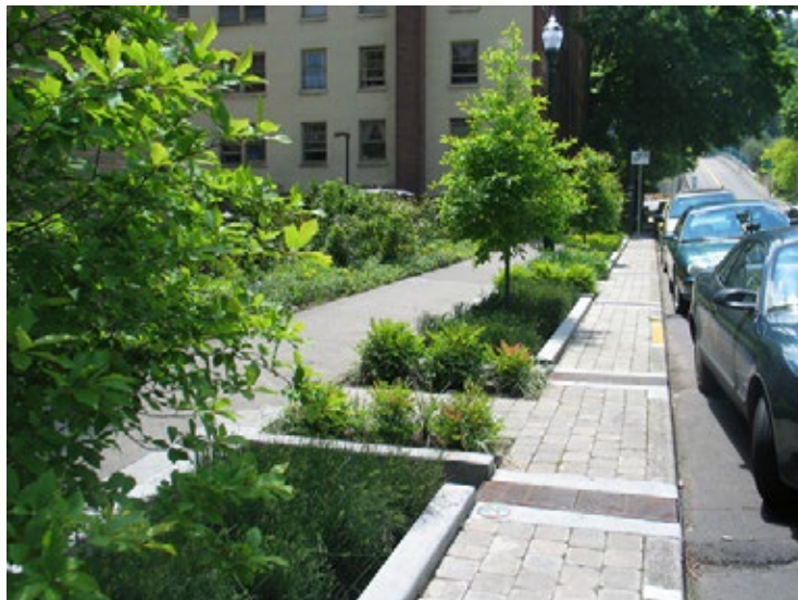
Sidewalk planters are equipped with bridges to provides access to parking areas in Seattle, WA.
