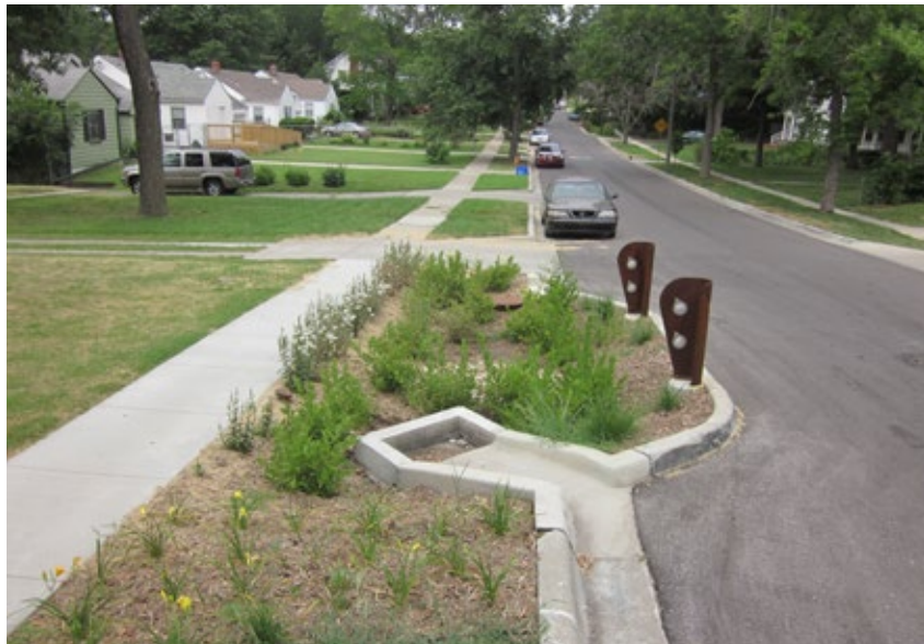
Mid-street stormwater curb extension in a neighborhood in Kansas City, MO.
