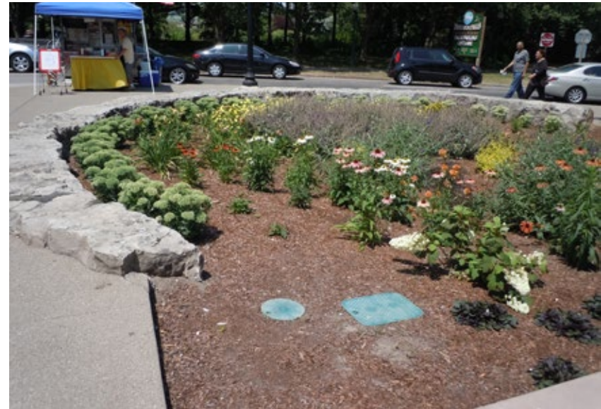
Bioretention in sidewalk with protective stone wall that doubles as a bench in Washington, DC.
