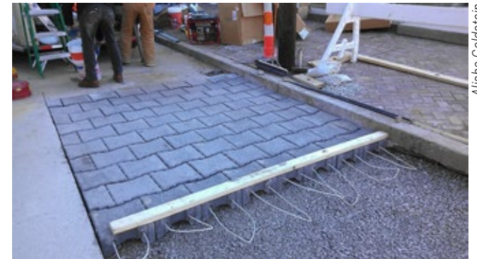
Permeable paver installation in parking lanes in Louisville, KY.
