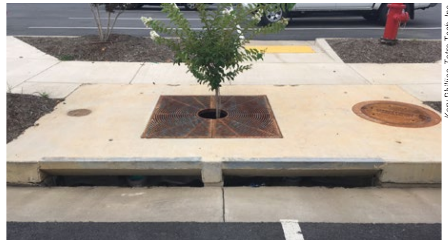
Stormwater catch basin tree pit, Charlottesville, VA.
