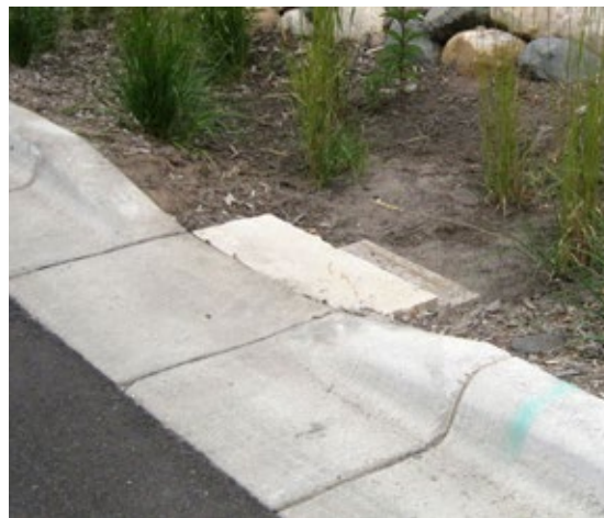
Figure 4-26. A wide-angled curb cut with an energy-dissipating splashpad also serves as access steps for maintenance in Maplewood, MN.
