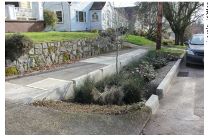
Curb cuts in the sidewalk and street allow for runoff to flow into this stormwater planter in Portland, OR.
