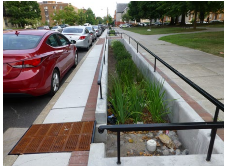
A pedestrian-friendly sidewalk planter includes safety rails and a metal sidewalk bridge in Baltimore, MD.
