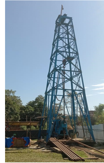
New BH south of the Highway being drilled
