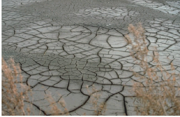
Figure 7 - Sludge in infiltration pond
