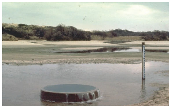
Figure 6 - Infiltration pond (drying up)
